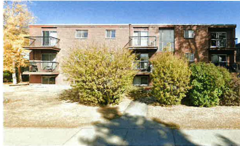
2136 4 AV NW, 240m east of WH405 (2.5 storey multi-residential in established low density residential area)
