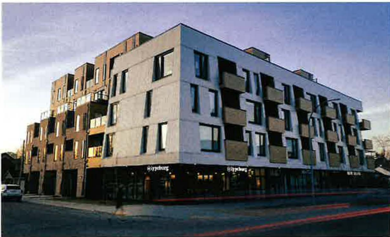
Hillhurst Manor (5 storey mixed-use multi-residential), 125m south of WH405 on 19 ST NW
