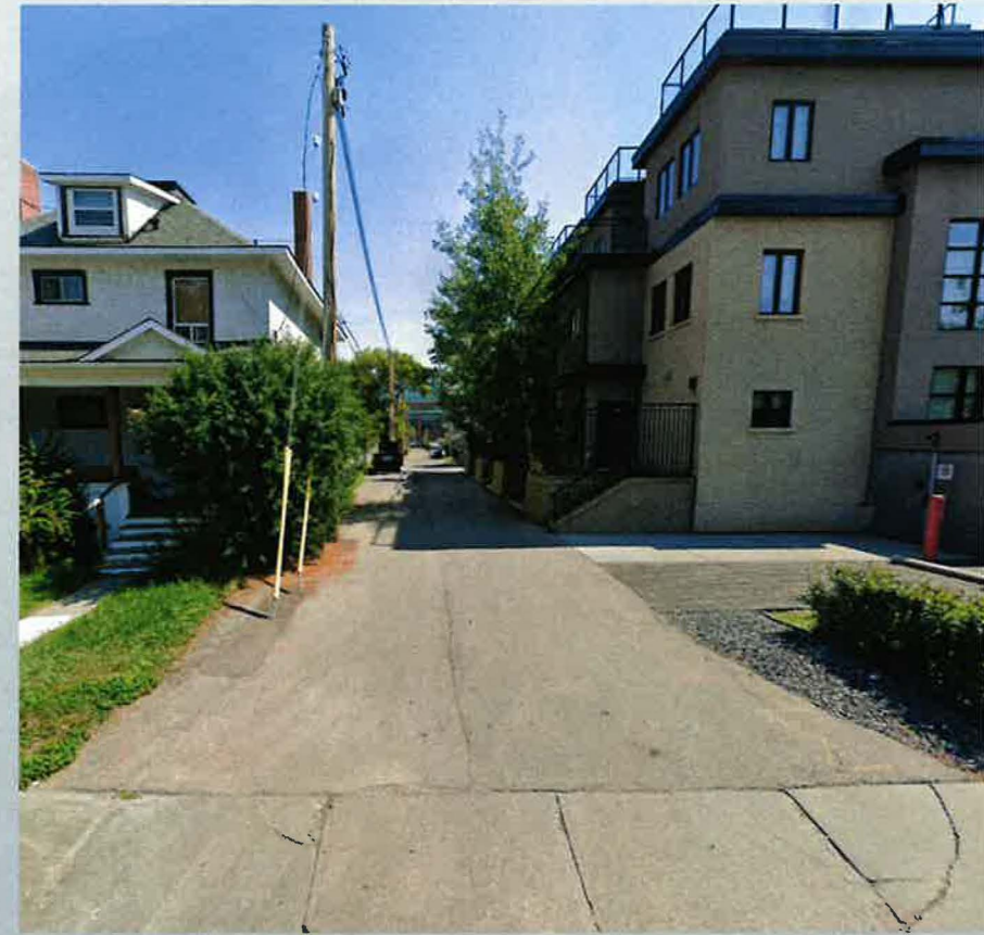
Existing lane condition with townhouse buildings on the south side
