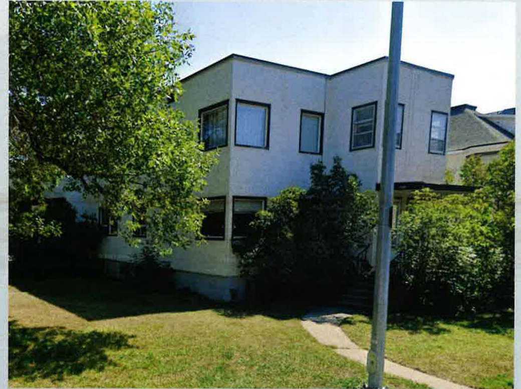
Existing apartment building on corner of 5 ST SW and 20 AVE SW
