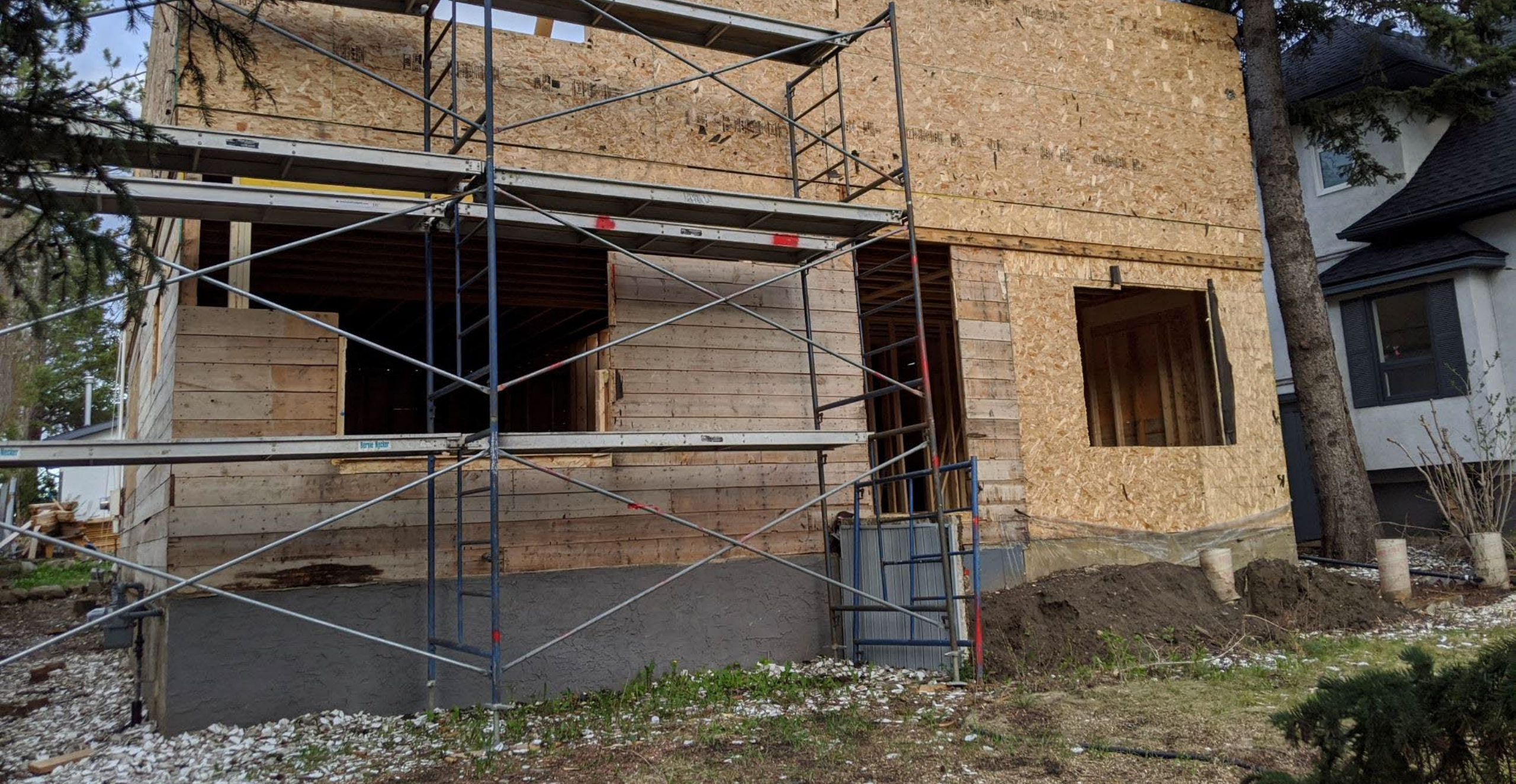
GRAHAM HOUSE, UNDER CONSTRUCTION, BRITANNIA
