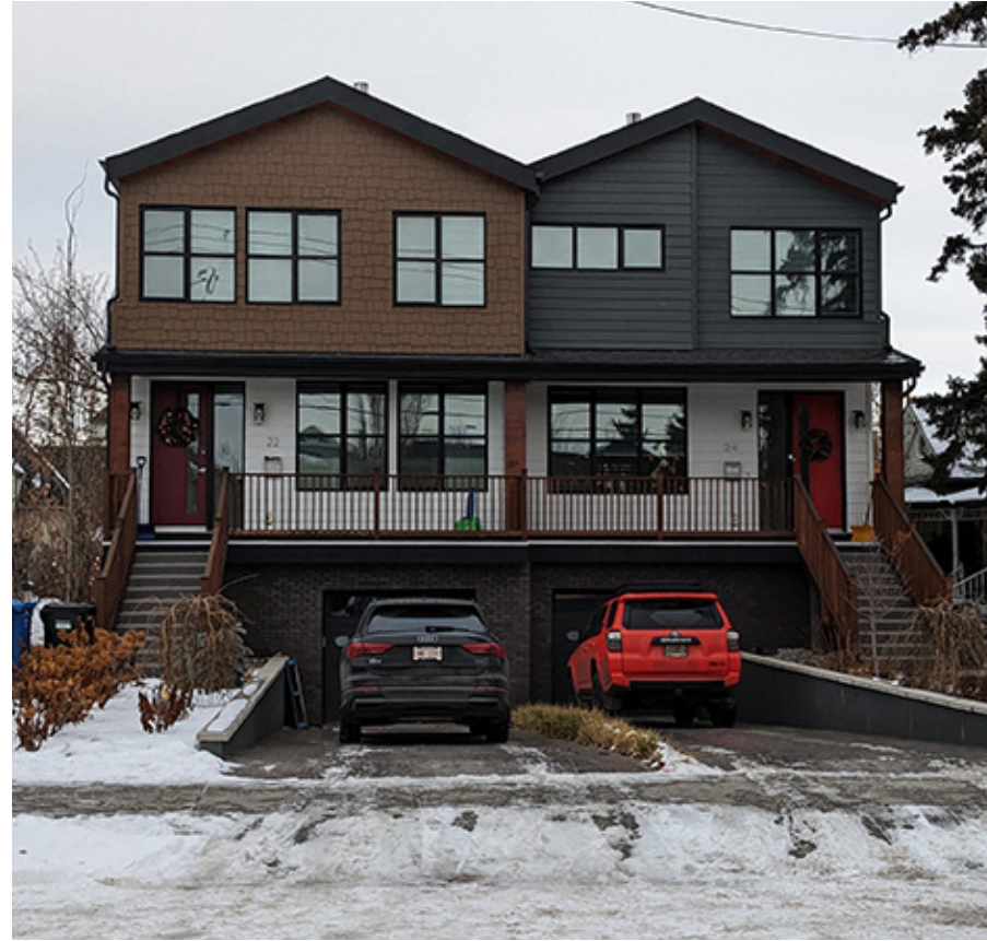
22 + 24 NEW STREET SE (TO THE WEST ON NEW STREET)
