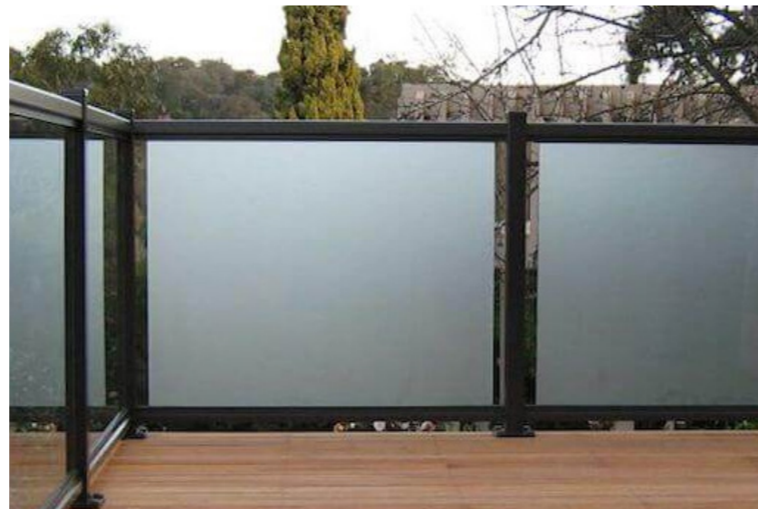
Balcony Guardrail Dark Grey Metal, Frosted Glass
