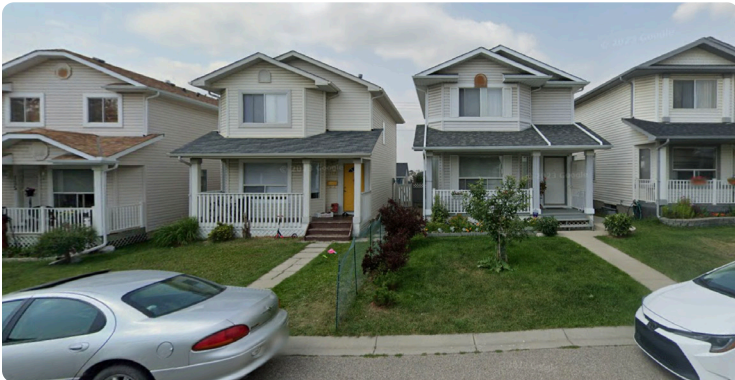
Existing Homes Arbour Wood Mews NW
