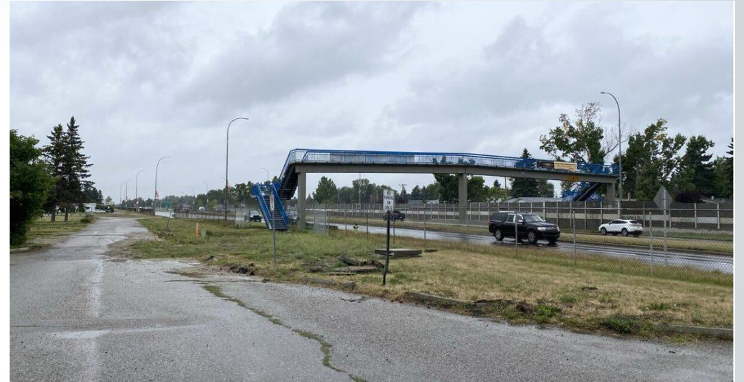
Existing Pedestrian Bridge over Blackfoot Trail.
