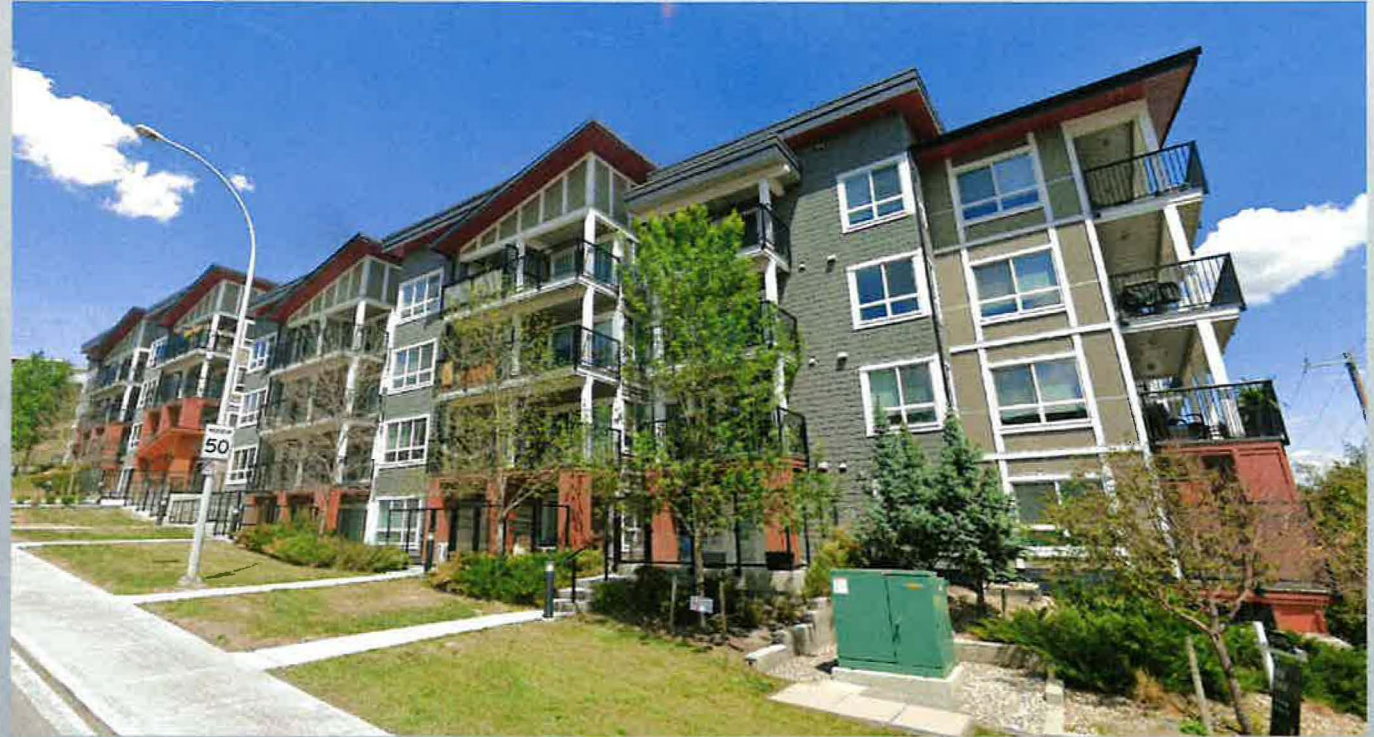
4 storey residential development at 510 Edmonton Trail NE (Bridgeland Hill)
