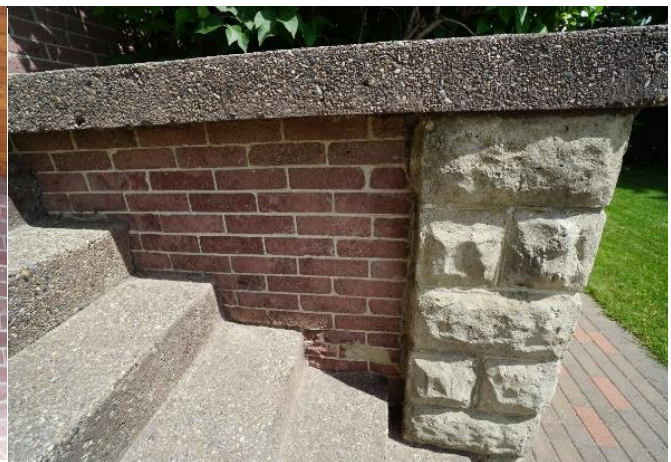
(Image 1.8: Detail showing exterior front stairs: walls of concrete bricks laid in stretcher bond and hollow rock-faced concrete blocks)
