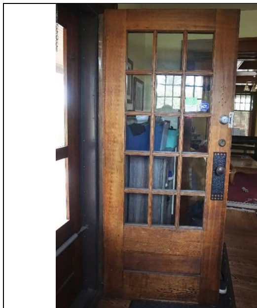
(Image 7.1 Main entry 15-pane Douglas fir door)
