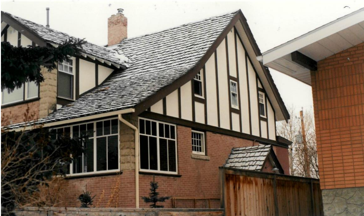
(Image 2.3: photo ca.1996, view of house from southeast)
