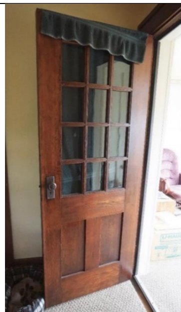
(Image 7.2 Second storey veranda 12-pane Douglas fir exterior door)
