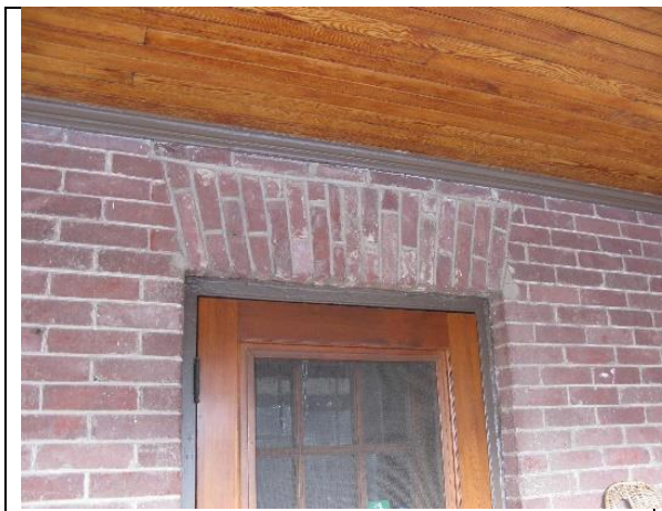
(Image 1.7: doorway with flat gauge lintel in concrete brick)
