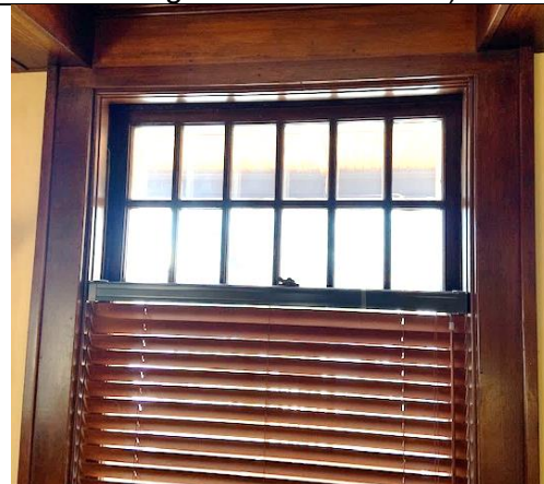
(Image 7.2 Second storey veranda 12-pane Douglas fir exterior door)
