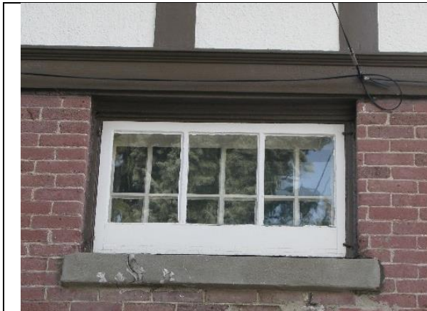
(Image 4.3: 12-pane wood window with concrete sill)
