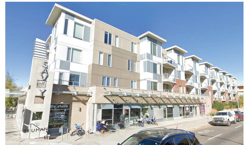
Savoy (4 storey mixed-use multi-residential), 250m south of WH405 on 19 ST NW
