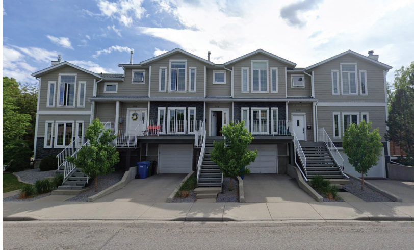
302 20 ST NW, 125m southeast of WH405 (3 storey rowhouse in established low density residential area)
