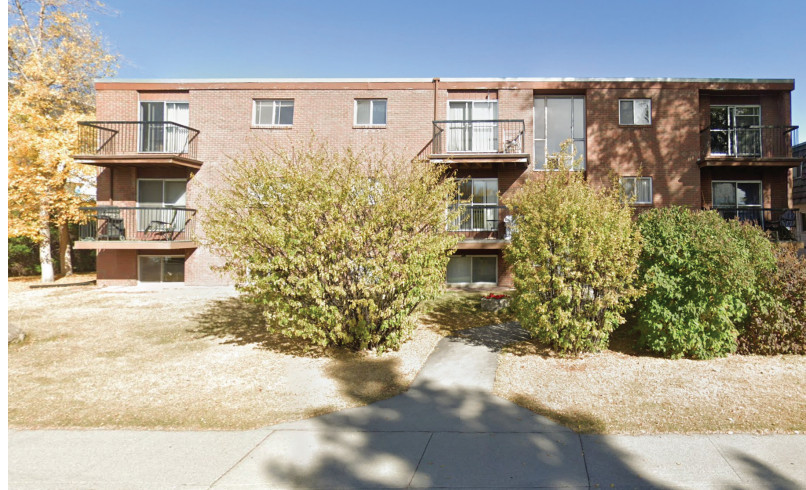
2136 4 AV NW, 240m east of WH405 (2.5 storey multi-residential in established low density residential area)
