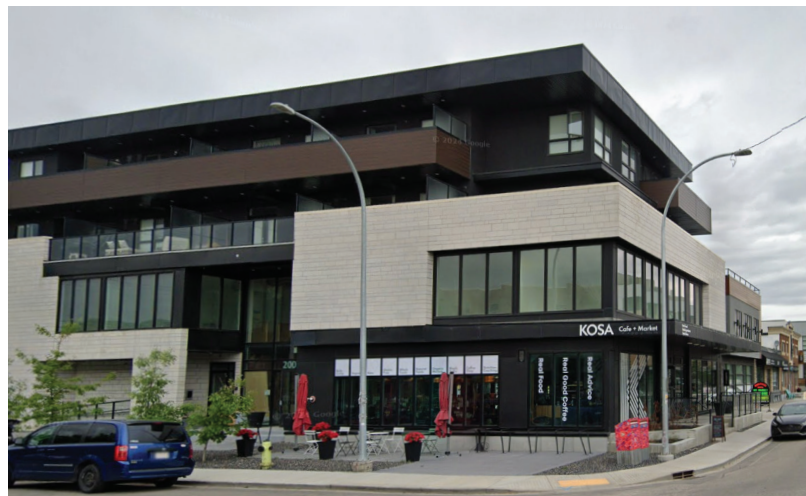
Wolf Den (4 storey mixed-use multi-residential), 210m south of WH405 on 19 ST NW
