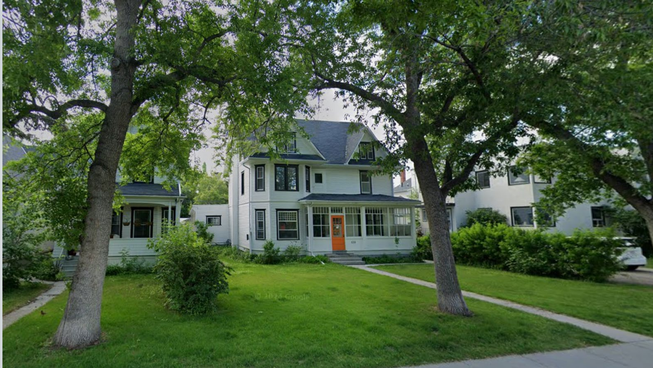
Existing single-detached dwelling that contain multiple units
