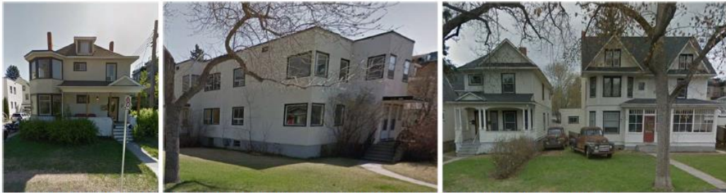
Figure 12. Four character homes are at risk of loss with respect to the Davis Block development in 2024
