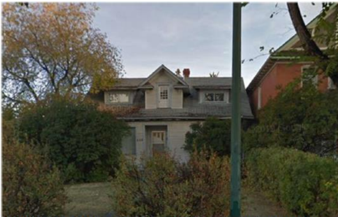
Figure 17. One character homes was demolished to develop a townhouse at 2298 5 Street SW in 2021
