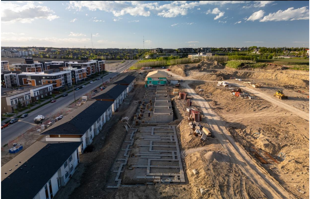
For sites located east of 77 St SW between 17 th Ave SW and 26 th Ave SW, grade-oriented townhouse and rowhouse buildings should not exceed three storeys
