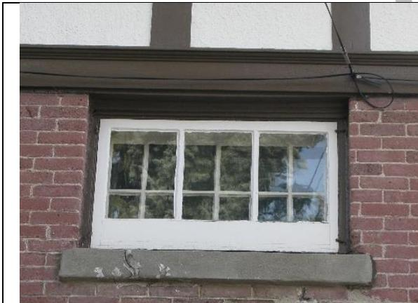
(Image 4.3: 12-pane wood window with concrete sill)
