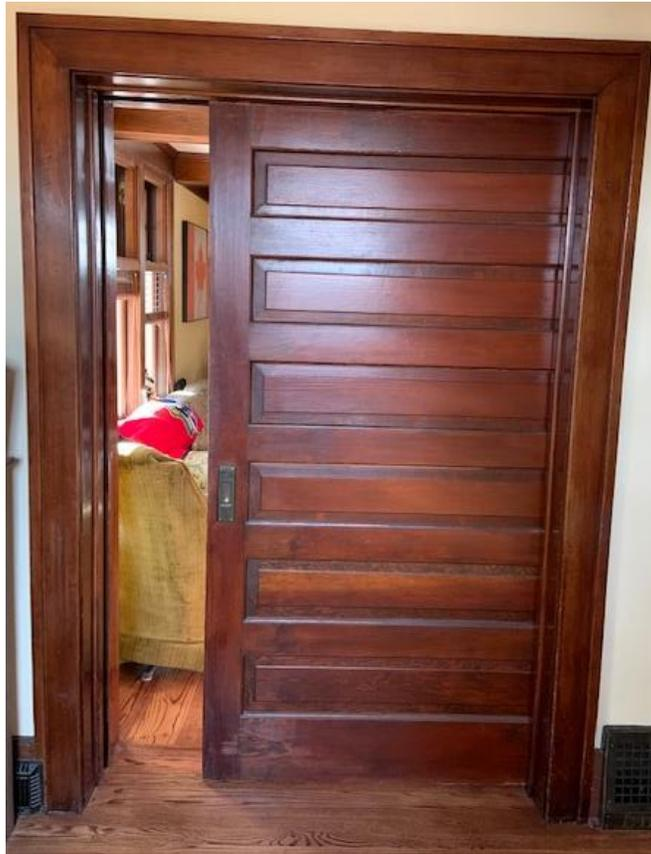
(Image 7.5 Pocket door and example of typical door casing)
