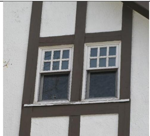
(Image 3.4: example of one of two double assemblies of 6-over-1 pane hung wood windows, with flat head and painted wood trim)
