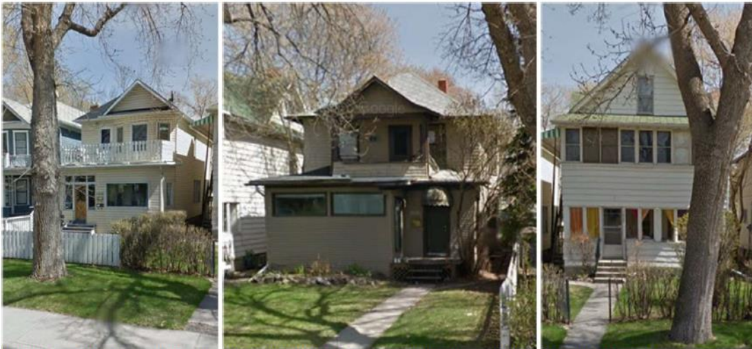
Figure 16. Three character homes were demolished to develop a townhouse at 1920 5A Street SW in 2015
