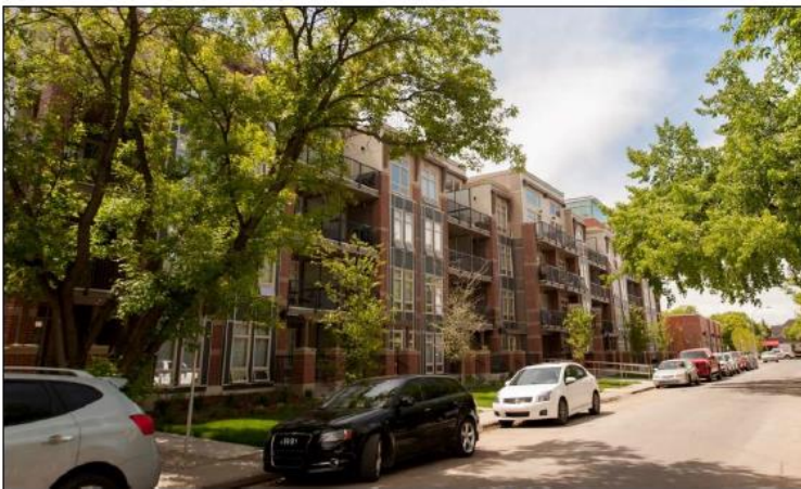
Figure 11: Bucci's Tribeca Condos, located in Cliff Bungalow-Mission at 323 20 Avenue SW
