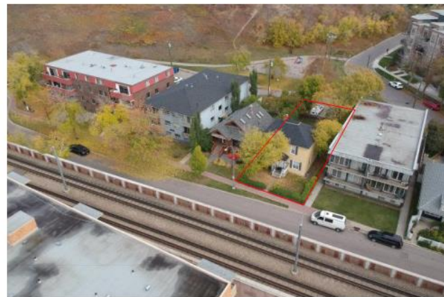
SW Site Corner
