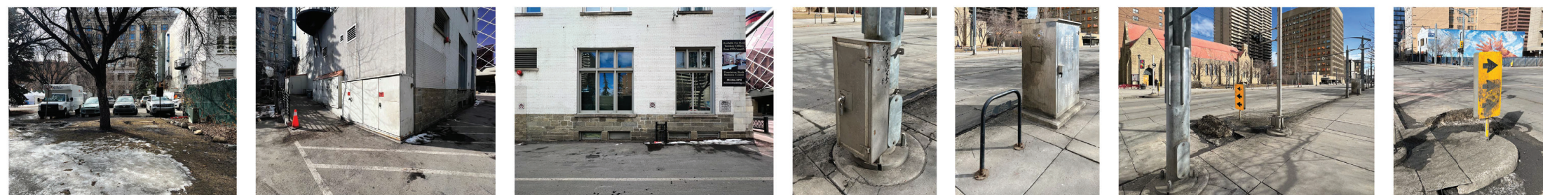
14 SITE PHOTO NORTH VIEW OF PARKING AT DOMINION BANK BUILDING NTS 13 SITE PHOTO VIEW OF UTILITY CABINETS ON NORTH EAST OF DOMINION BANK BUILDING NTS 12 SITE PHOTO DIRECT VIEW OF DOMINION BANK BUILDING FROM NORTH NTS 11 SITE PHOTO VIEW OF LEFT UTILITY BOXES NTS 10 SITE PHOTO VIEW OF LEFT UTILITY BOXES NTS 9 SITE PHOTO VIEW OF CURB AT LEFT LINE FROM SOUTH WEST NTS 8 SITE PHOTO VIEW OF CURB AT LEFT LINE FROM SOUTH EAST NTS
