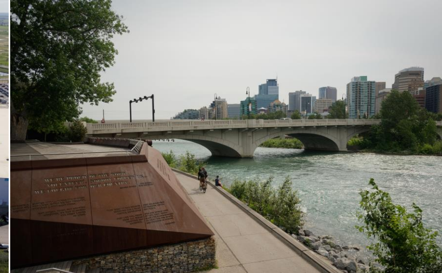
Building a 1:100 level flood barrier to increase our flood resiliency
