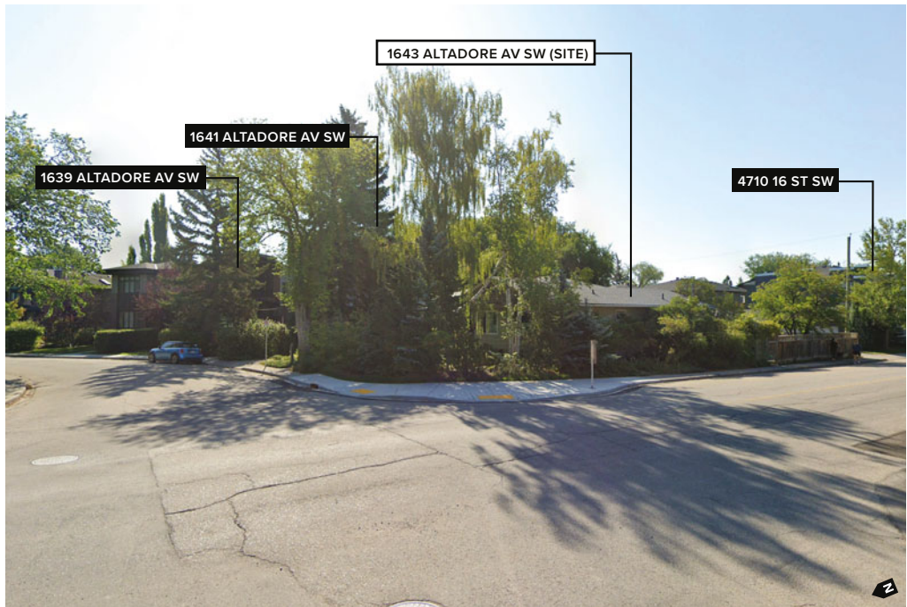
Looking southeast towards existing building and adjacent properties
