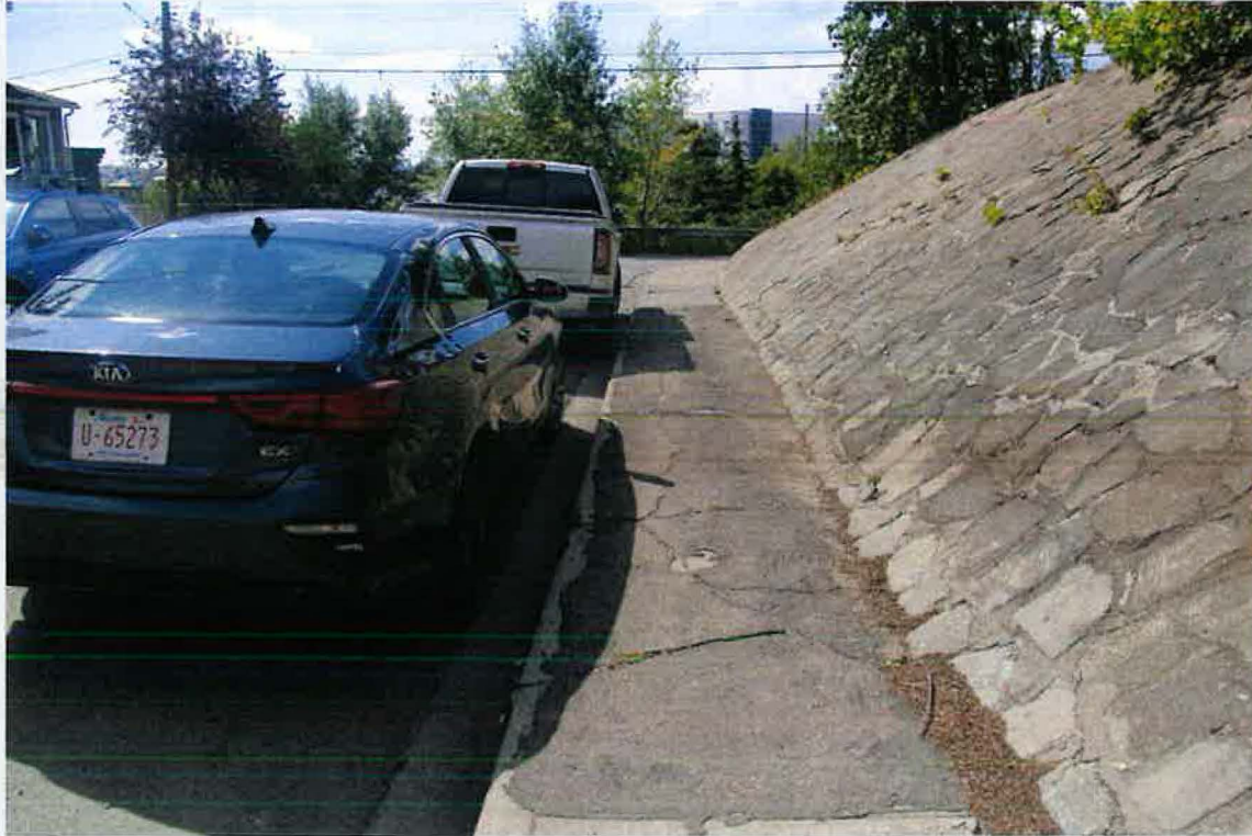
The dead-end of Erlton Court
