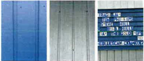
03 EXISTING BLUES CAN BUILDING MATERIALS
