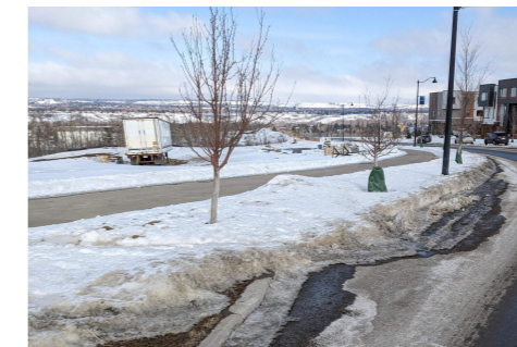
6. STREET VIEW OF CURB
