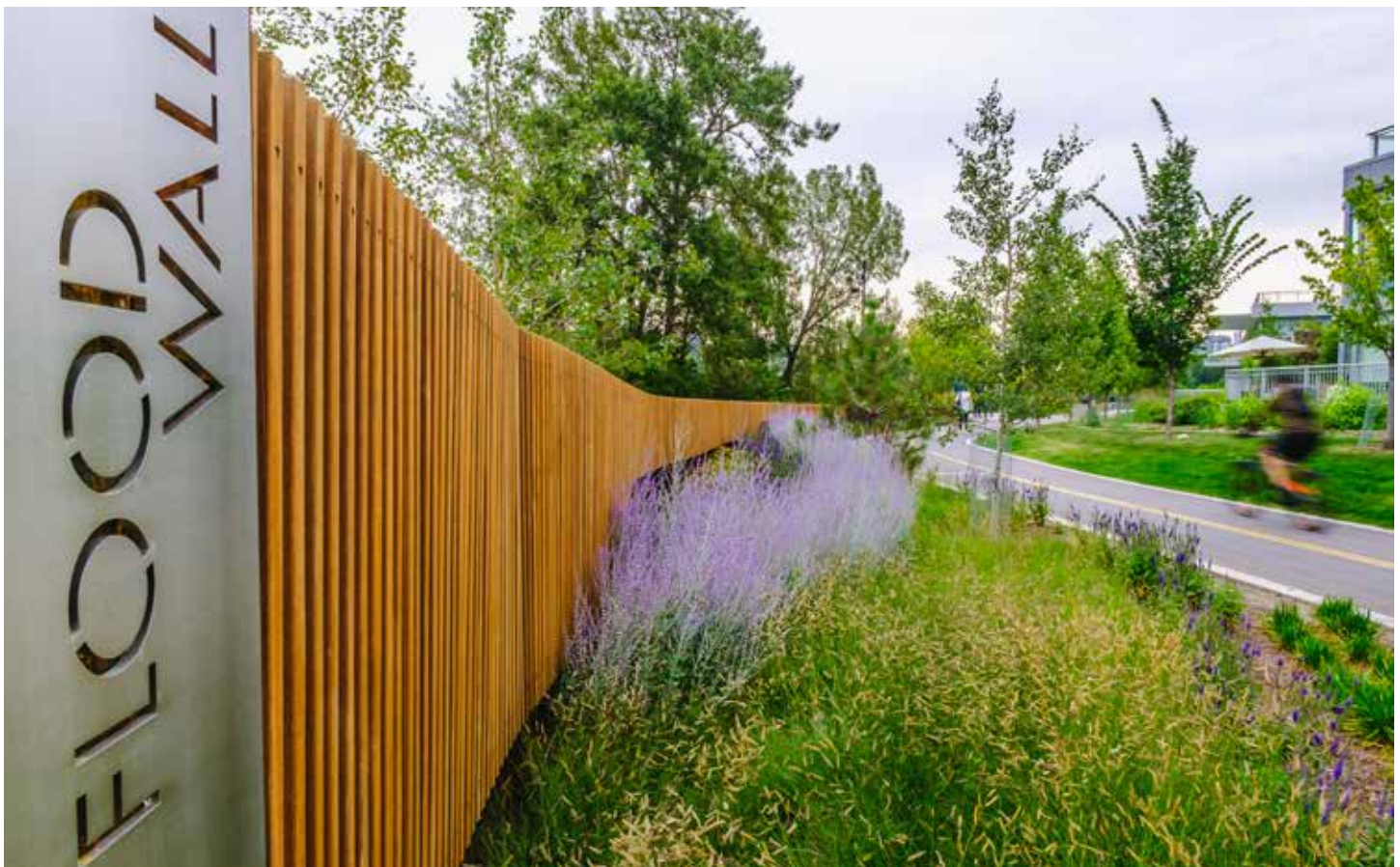
The Downtown Flood Barrier is 1.39km of steel sheet piles, earthen berms and concrete walls built to resist a 1:200 year flood event. ISC: Unrestricted
