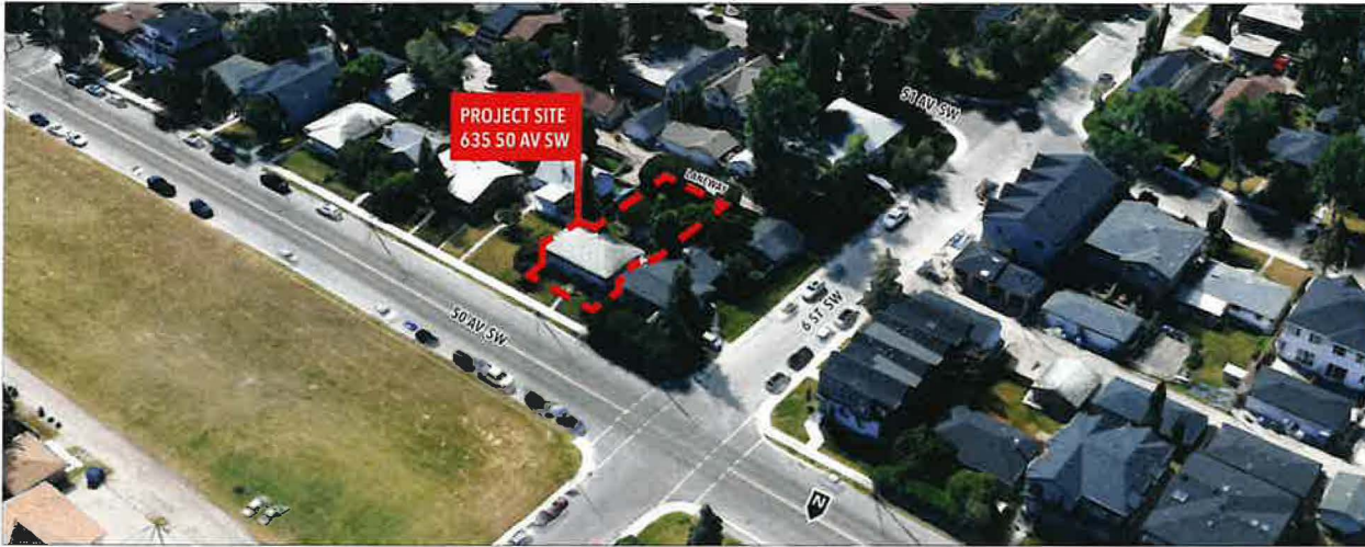
Subject Site – Aerial View
