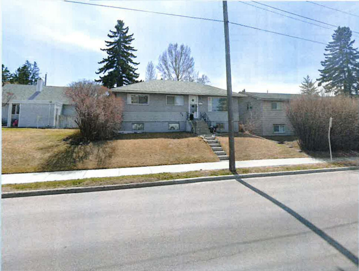
View from 50 Avenue SW
