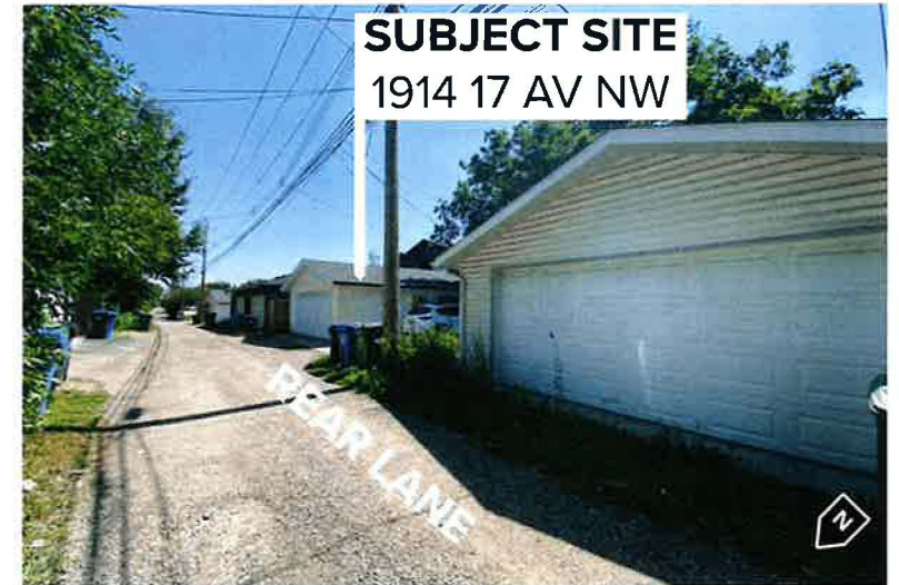
Looking Southwest from rear lane
