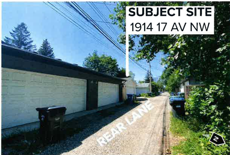
Looking Southwest from rear lane
