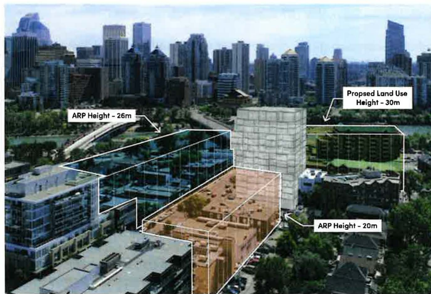
Figure 2: Applicant's Image Showing Surrounding Policy and Land Use Heights (not to scale)
