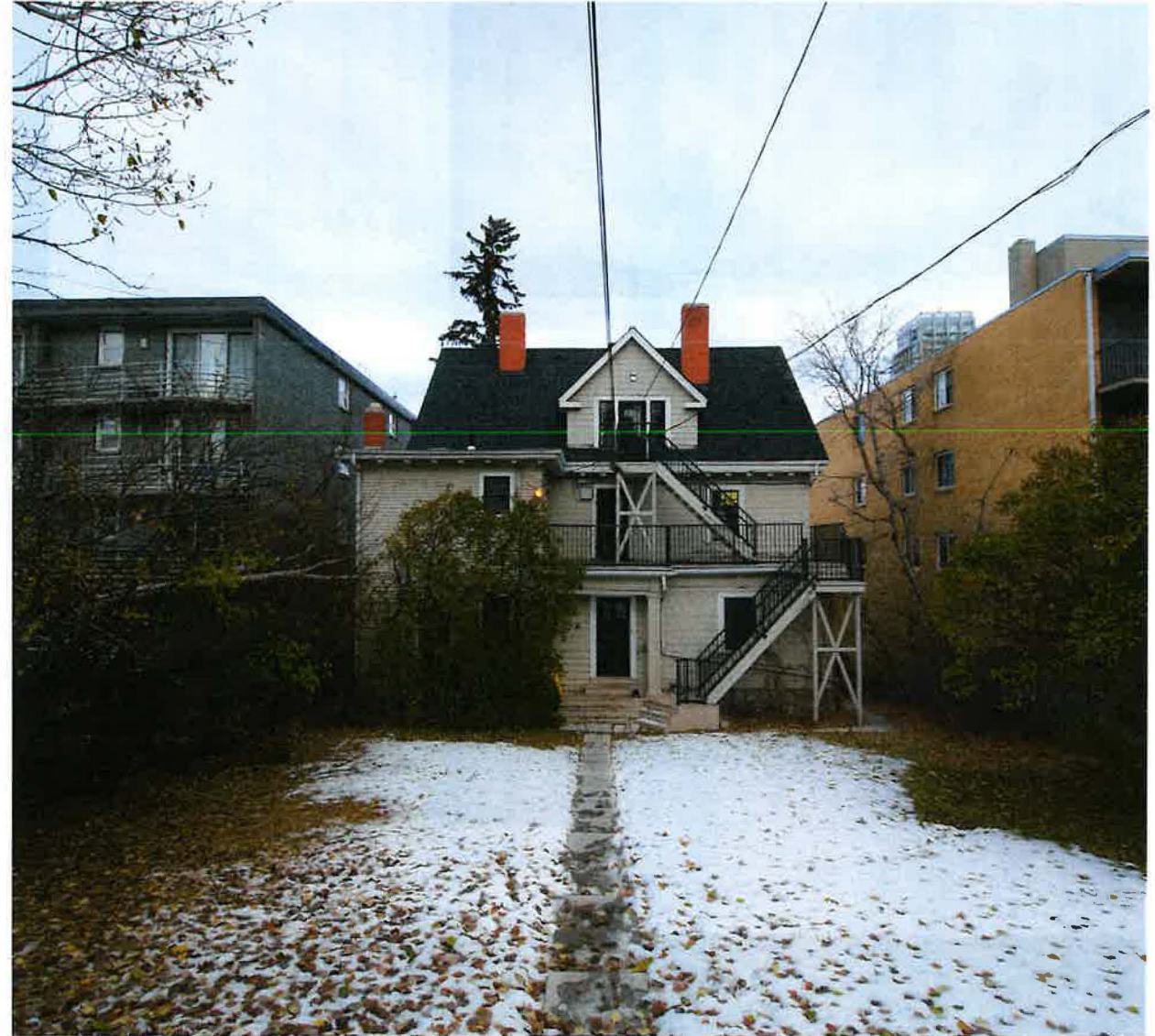
Looking South from Interior Yard near Royal AV SW
