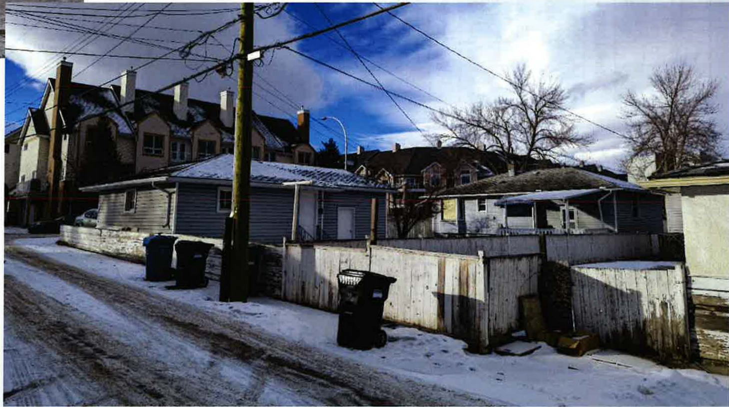
Rear view looking northwest
