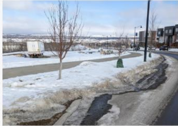
2. Street View of Curb
