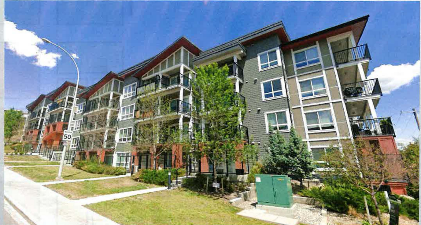
4 storey residential development at 510 Edmonton Trail NE (Bridgeland Hill)
