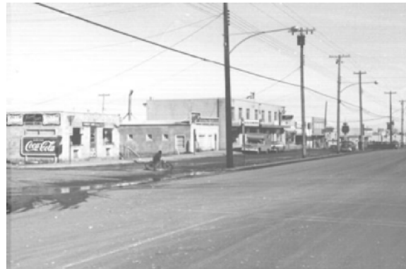
Photo: "17 Avenue SE Calgary, Alberta". Courtesy of International Avenue Business Revitalization Zone
