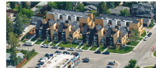
Example of a courtyard-oriented development on a larger site located two blocks to the south
