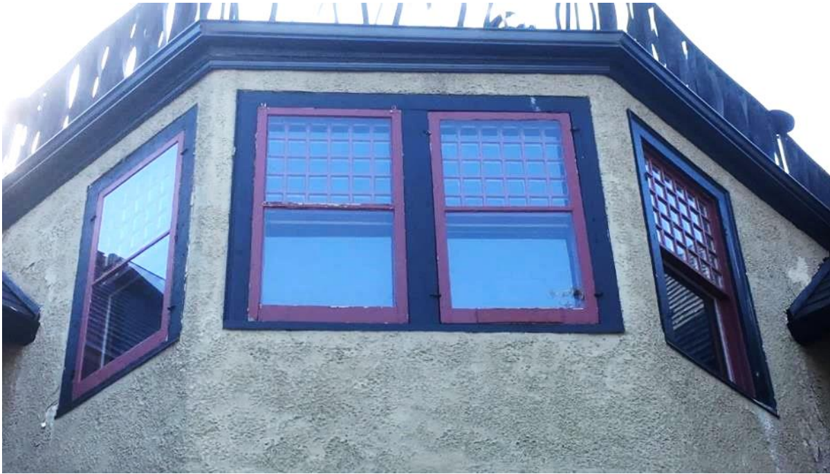
(Image 3.9: Example of original fenestration of multi-light-over-single pane wood windows and casings. Note: Storm windows are not regulated)
