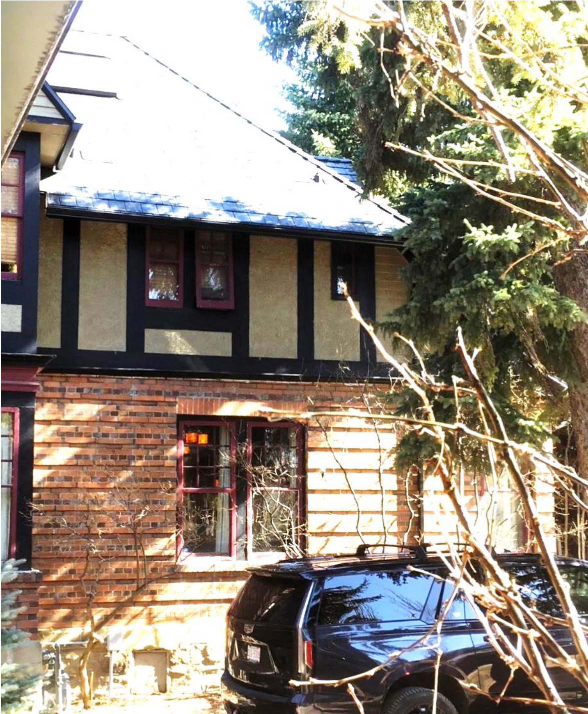
(Image 5.2: Southerly portion of west façade showing sandstone foundation, banded brick cladding (1 st storey), moulded wood cornice, rough-cast stucco and decorative wood half-timbering and shingles (2 nd storey) and fenestration. Note: Storm windows are not regulated)
