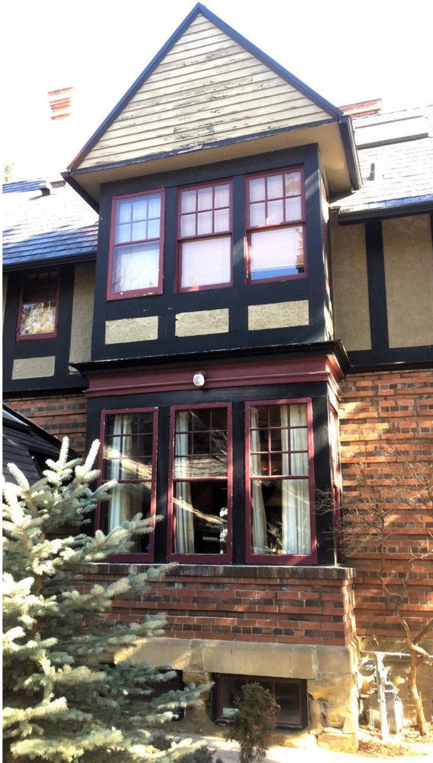
(Image 5.3: Close up of two-storey box bay window projection. Note: Storm windows are not regulated)
