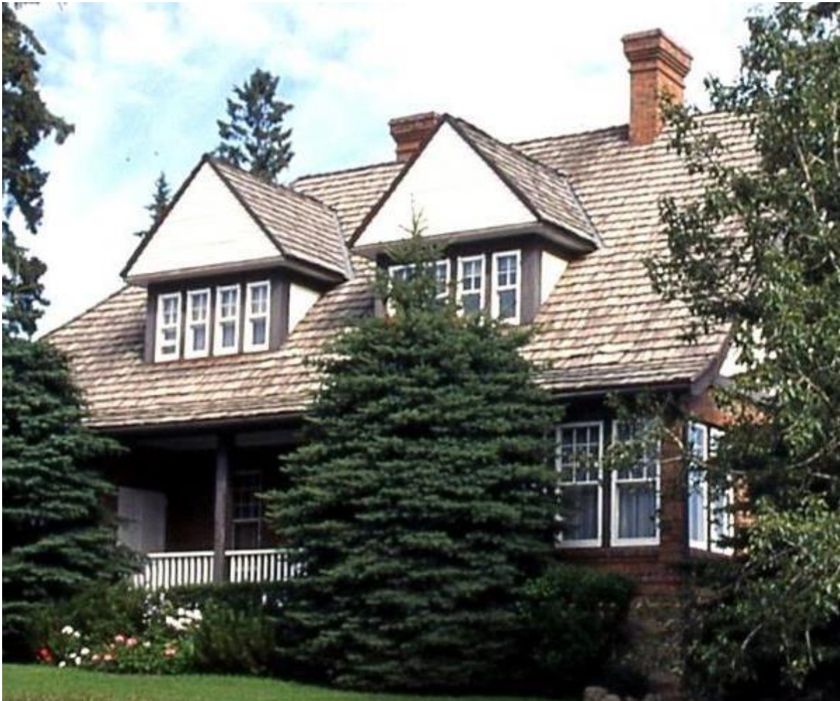
(Image 4.1: South façade ca. 1995 showing side-gable roof with flared bottom eave, inset porch and paired dormers)
