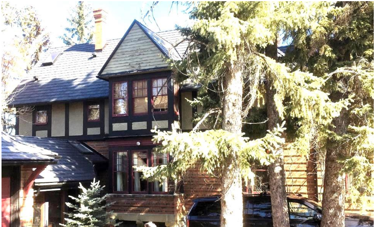
(Image 5.1: Northerly portion of west façade showing banded brick cladding (1 st storey), moulded wood cornice, rough-cast stucco and decorative wood half-timbering (2 nd storey) and fenestration. Note: Storm windows are not regulated)
