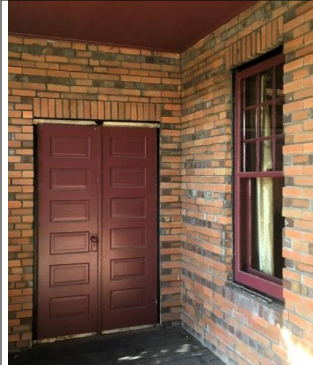
Image 4.2: Example of the paired, six-panel wood doors in the inset central porch (west side).
