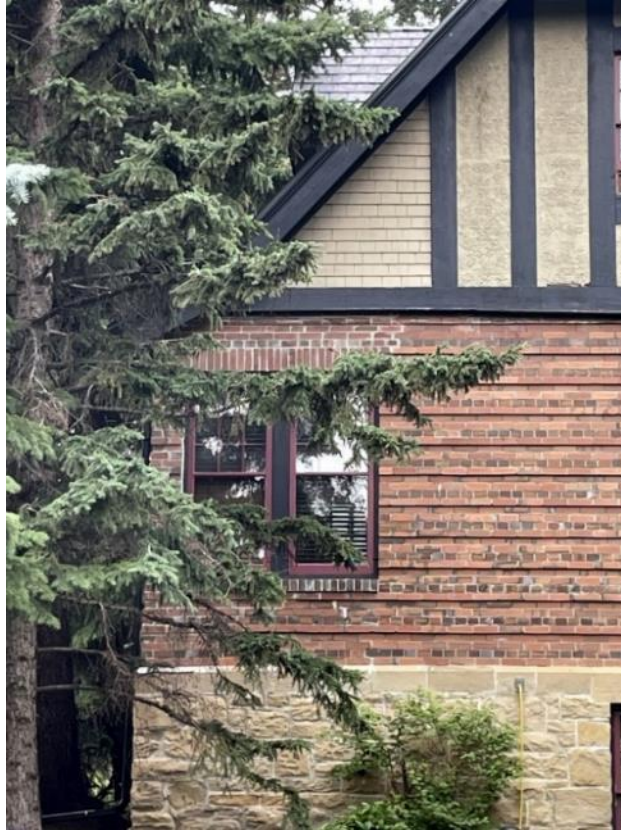
(Image 3.2: Portion of east façade showing typical random ashlar, cut sandstone foundation, banded brick cladding (1 st storey) and decorative wood half-timbering and shingles (2 nd storey).
