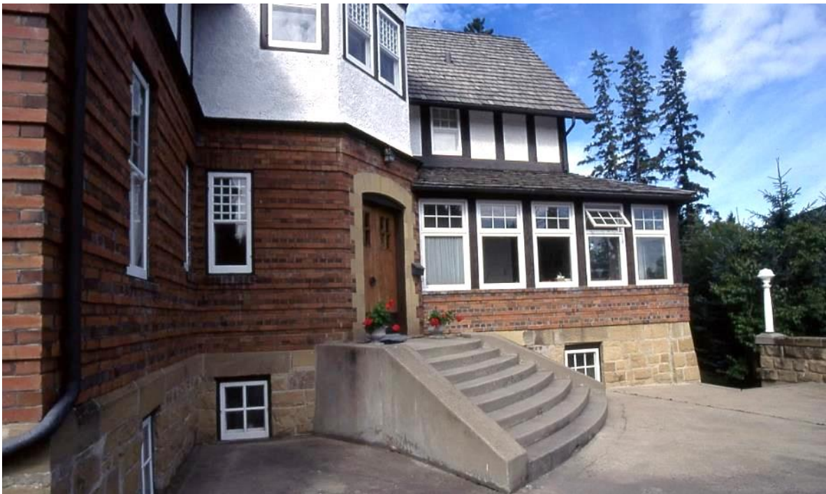
(Image 3.3: East façade ca. 1995 showing battered (sloped) north corner of sandstone foundation and main entry way tabbed with cut sandstone)
