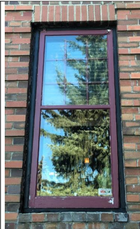
Image 3.8: Example of original fenestration with multi-light-over-single pane wood window with soldier course brick header and header course brick sill. Note: Storm window is not regulated.
