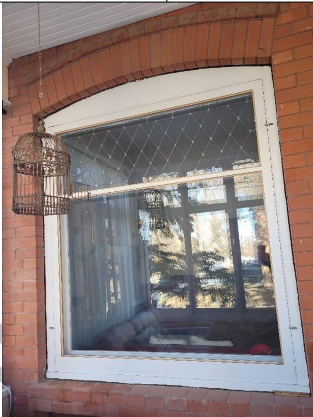
(Image 2.8: example of 1-over-1 window with decorative diamond patterned upper sash; segmental arch brick headers topped with rusticated course and protruding double course brick sills)
