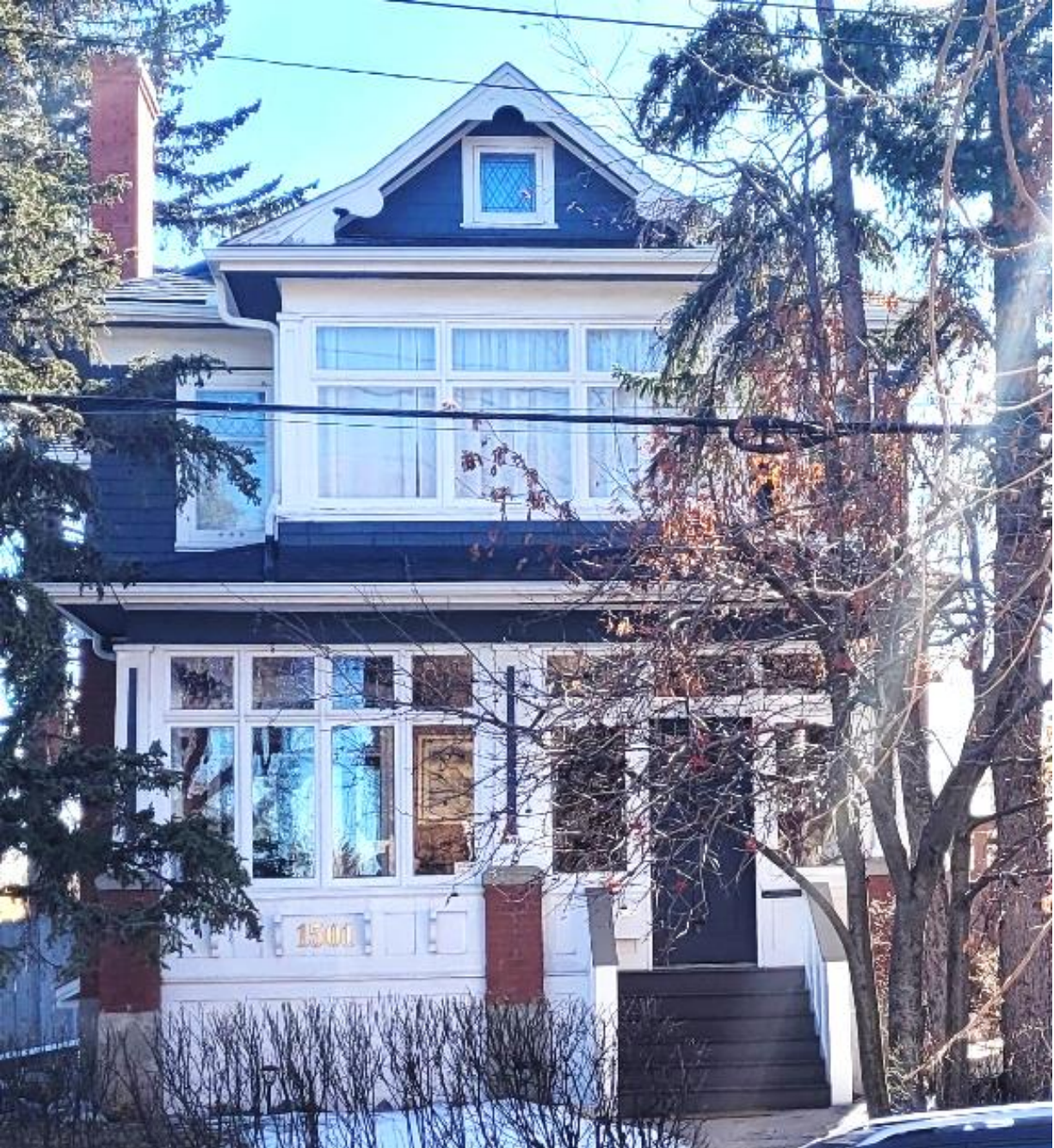
(Image 2.1: North façade)
