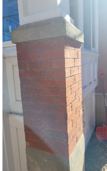
(Image 2.6: concrete and brick pedestals with stone caps)
