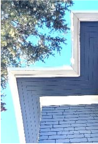
(Image 2.5: example of closed wooden tongue-and-groove soffits)
