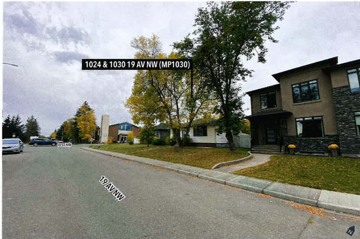
Looking north west at subject site from 19 AV NW
