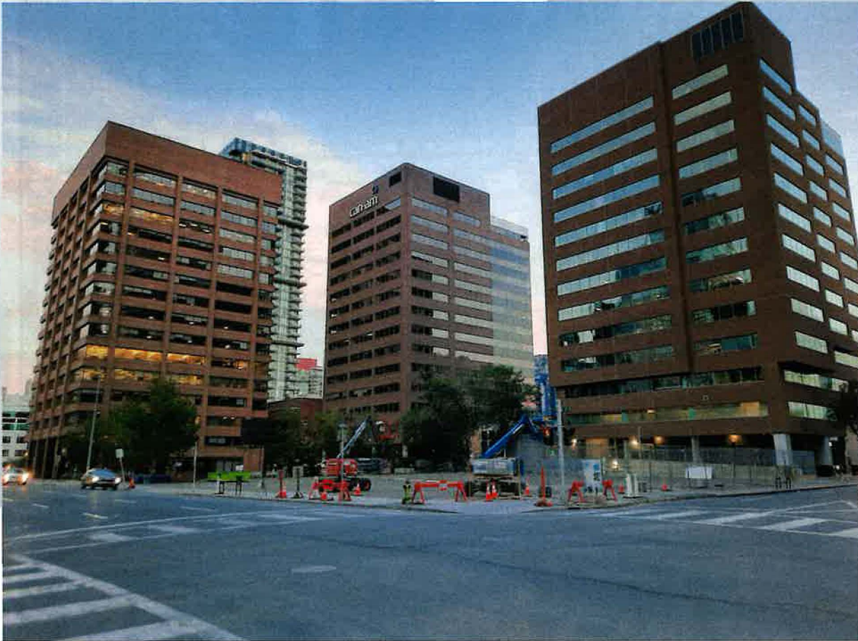
North-West Corner (11 Avenue SW & 4 Street SW)
