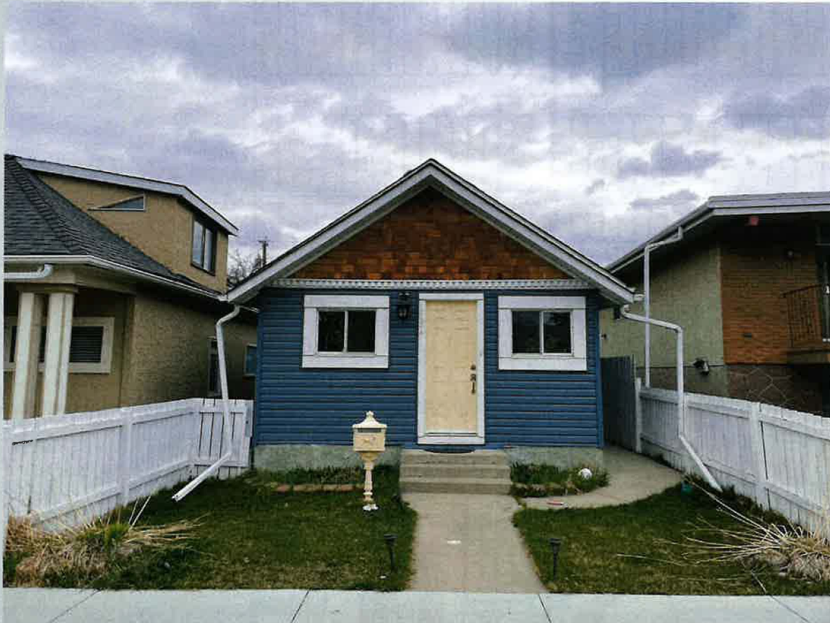
Looking north from 20 Avenue NW.
