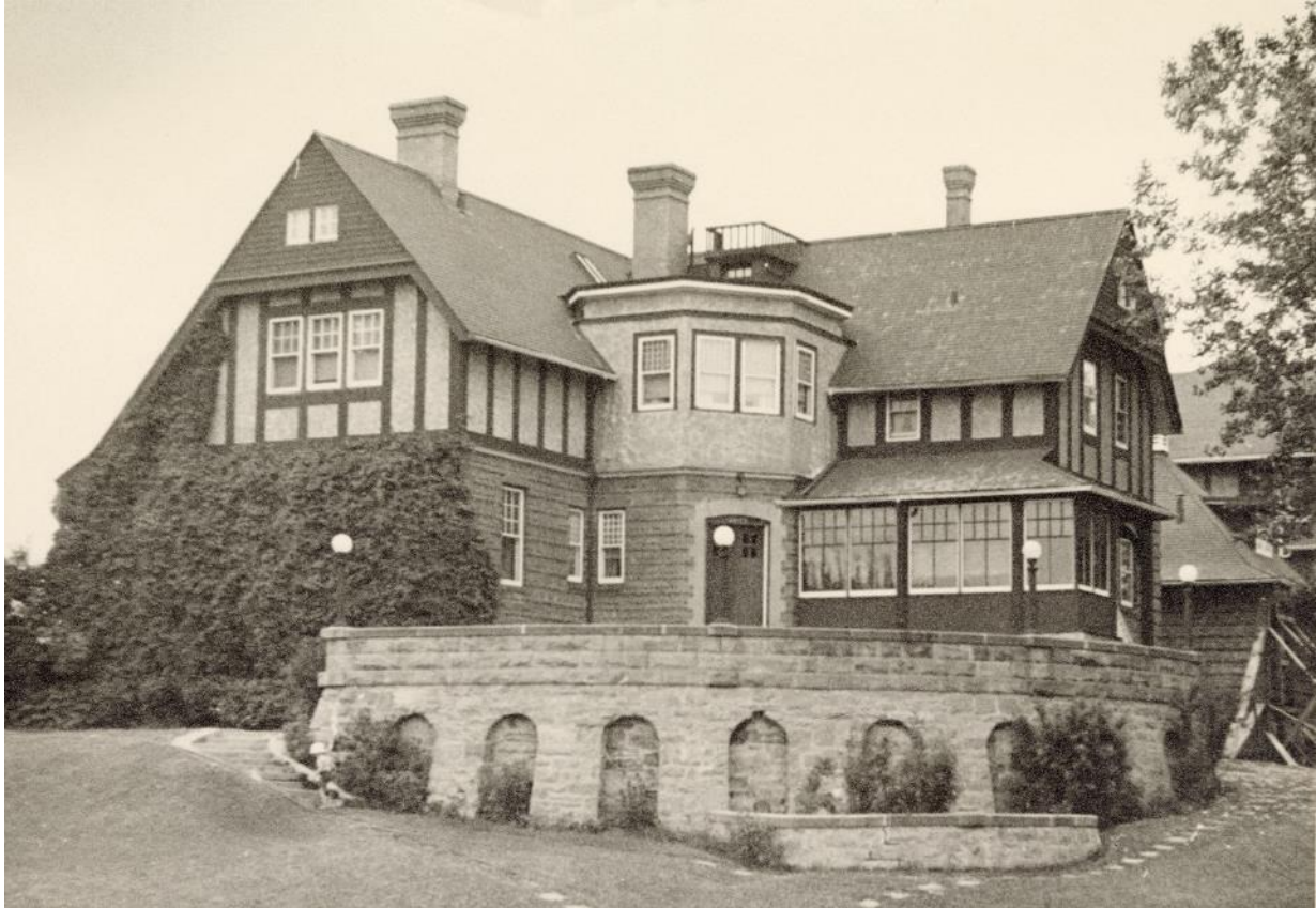
(Image 3.1: East and north façades ca. 1930 showing form, roof profile, cladding, fenestration and above grade, rounded terrace retaining wall - courtesy of Glenbow Library and Archives Collection (CU 1234217))
