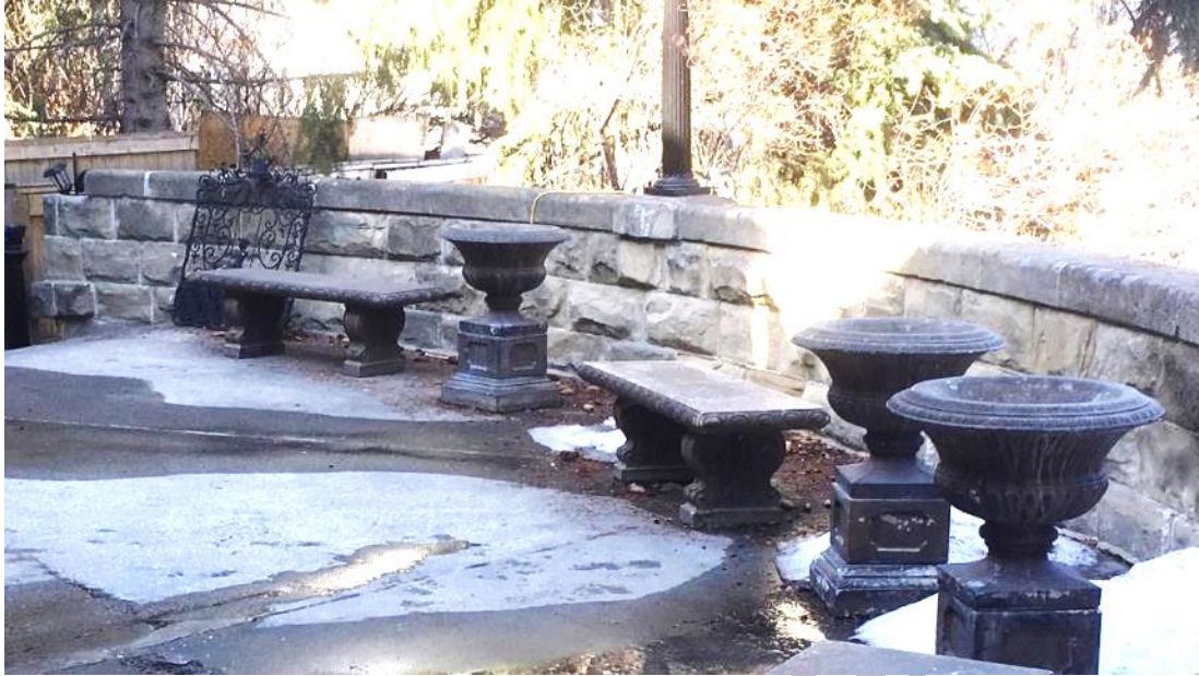
(Image 3.4: Interior of above grade, rounded terrace with cut sandstone balustrade and coping)
