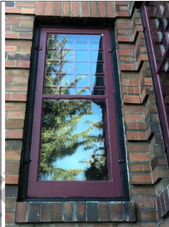
Image 3.7: Example of original fenestration with multi-light-over-single pane wood window with soldier course brick header and rowlock brick sill. Note: Storm window is not regulated.
