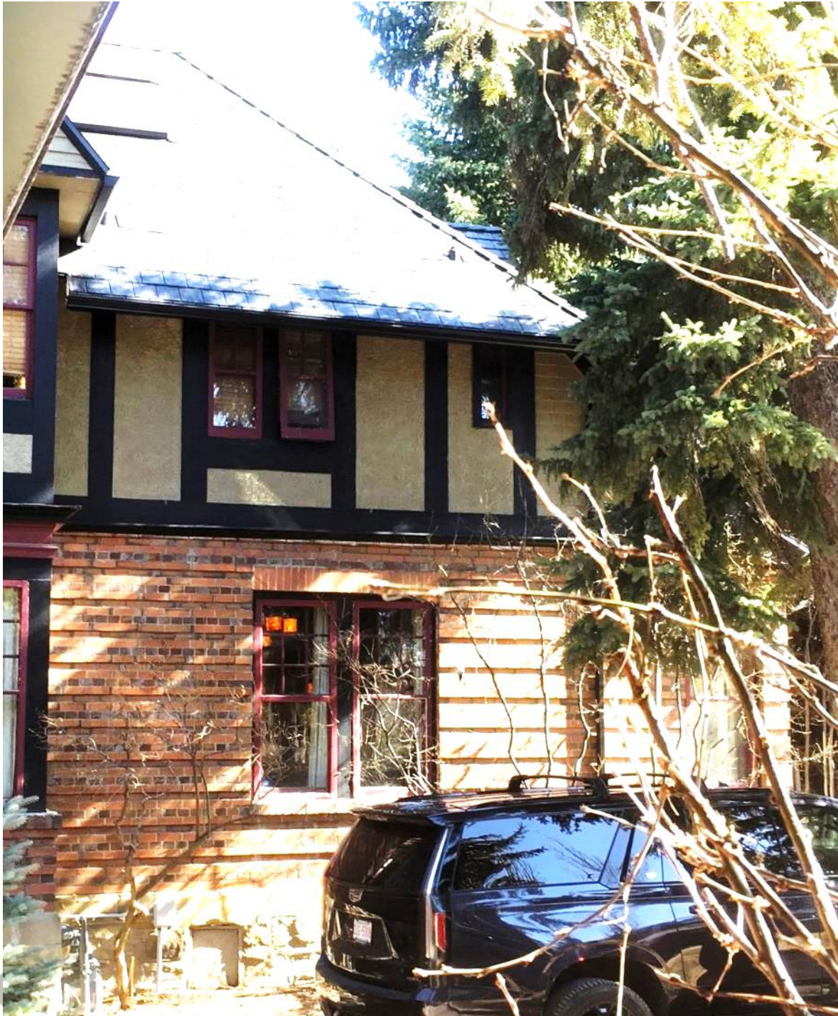
(Image 5.2: Southerly portion of west façade showing sandstone foundation, banded brick cladding (1 st storey), moulded wood cornice, rough-cast stucco and decorative wood half-timbering and shingles (2 nd storey) and fenestration. Note: Storm windows are not regulated)
