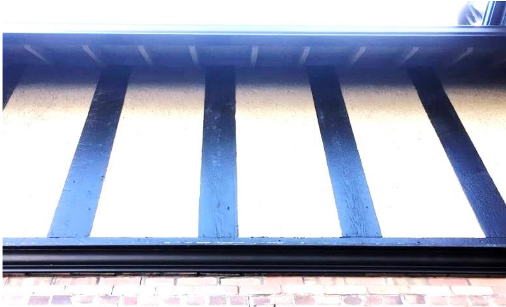
(Image 3.6: Close up of moulded wood cornice above brick cladding, decorative wood half-timbering and eaves with exposed rafters)
