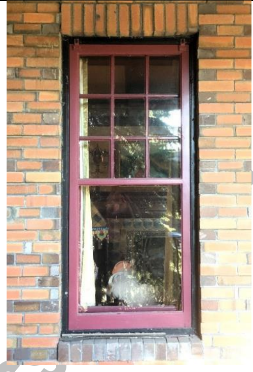
Image 4.3: Example of original fenestration of multi-light-over-single pane window with soldier course brick header and rowlock course brick sill. Note: Storm window is not regulated.
