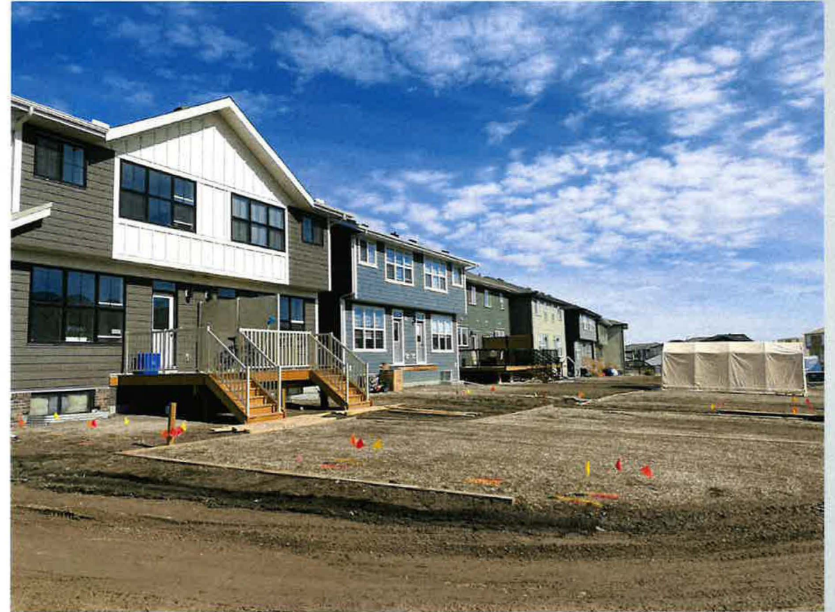
Location from the rear lane facing northeast
