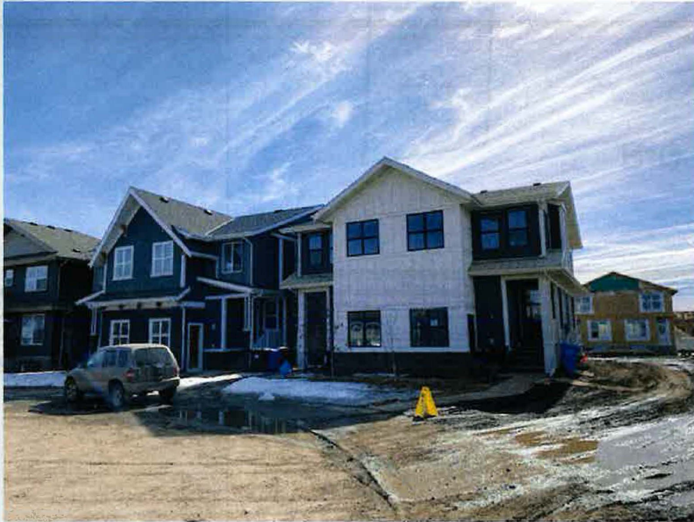
View towards the subject site
