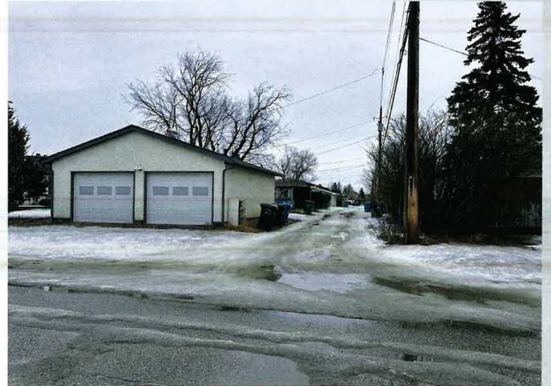
View of the subject site looking east
