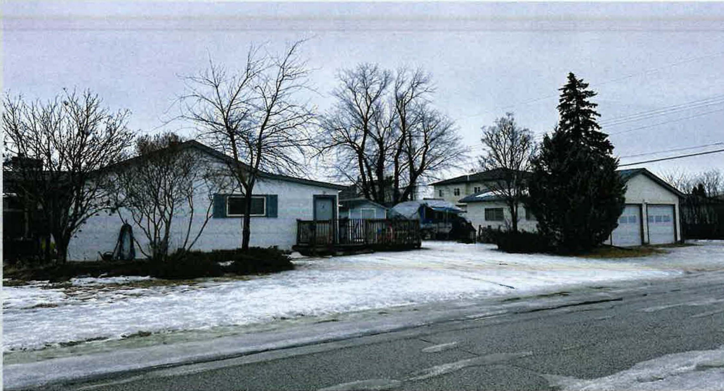
View of the subject site looking southeast
