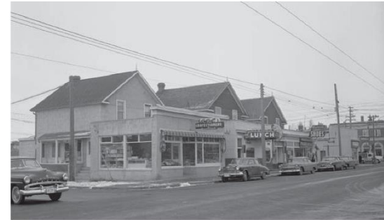
Shops built in front of older homes along 14 Street SW, looking southeast toward 17 Avenue, 1956. Jack De Lorme, photographer. Glenbow Library and Archives Collection, Libraries and Cultural Resources Digital Collections, University of Calgary, CU1140020
