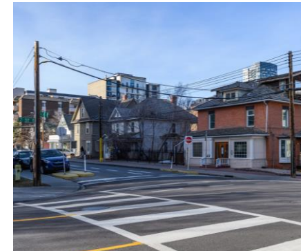
Shallow Utility Relocation Program
