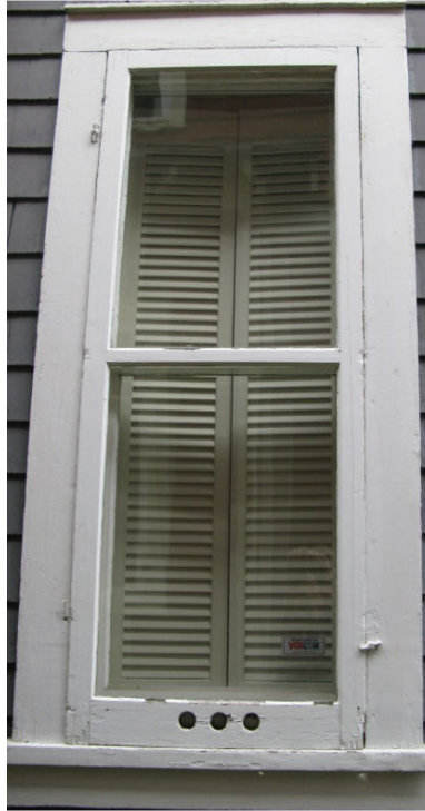
(Photo 1.4: an example of a wooden-sash window and casings)
