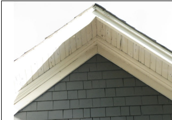
(Photo 5.1: an example of the wooden soffits and cornice/frieze mouldings)
