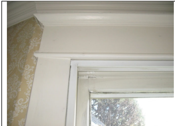
(Photo 6.4: an example of the window casings – upper portion)
