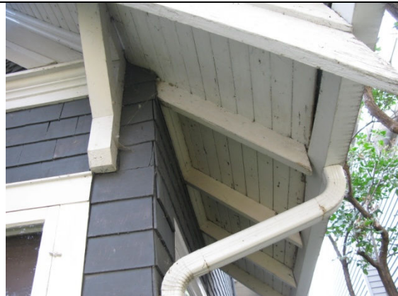
(Photo 5.2: and example of the exposed rafter tails, extended bargeboards and triangular brackets)
