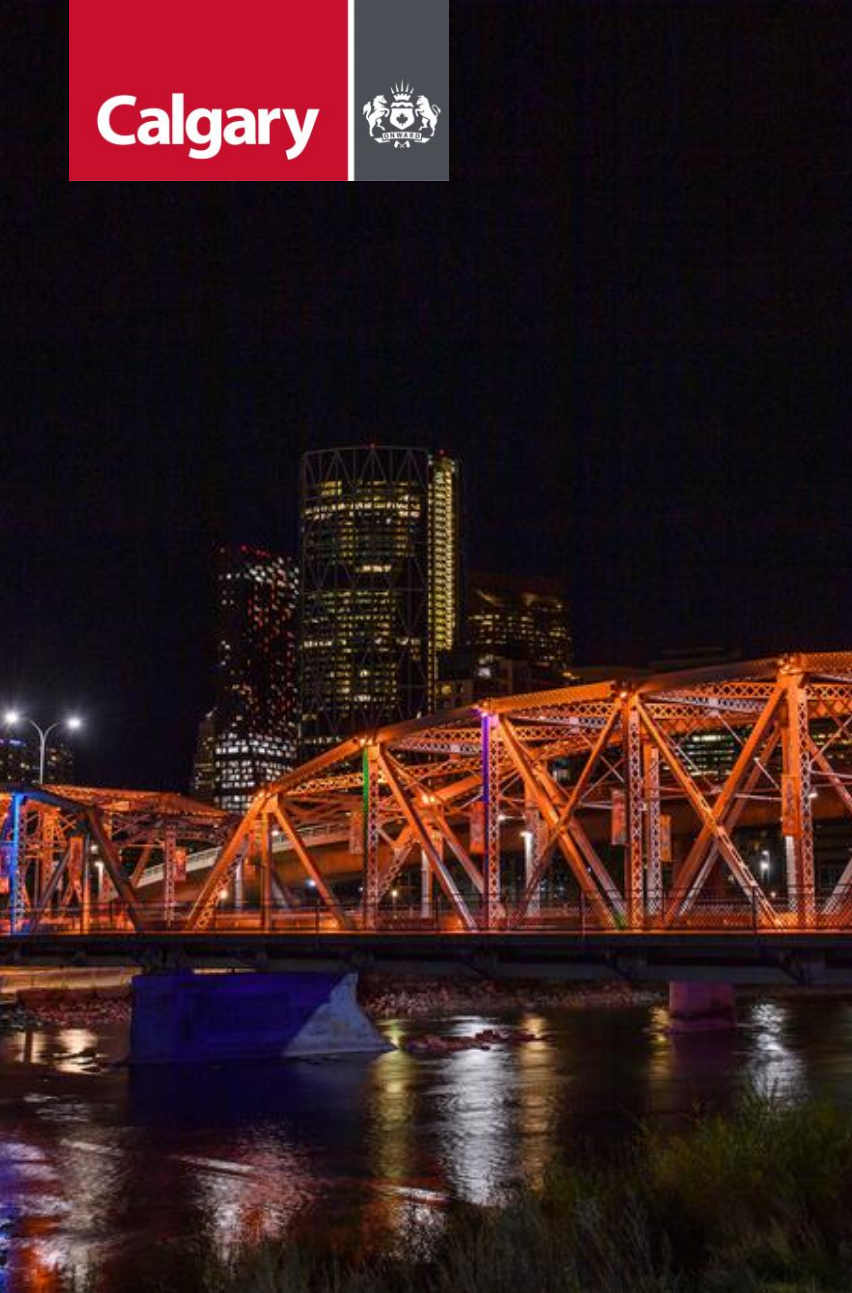
Langevin Bridge renamed to Reconciliation Bridge in 2017
