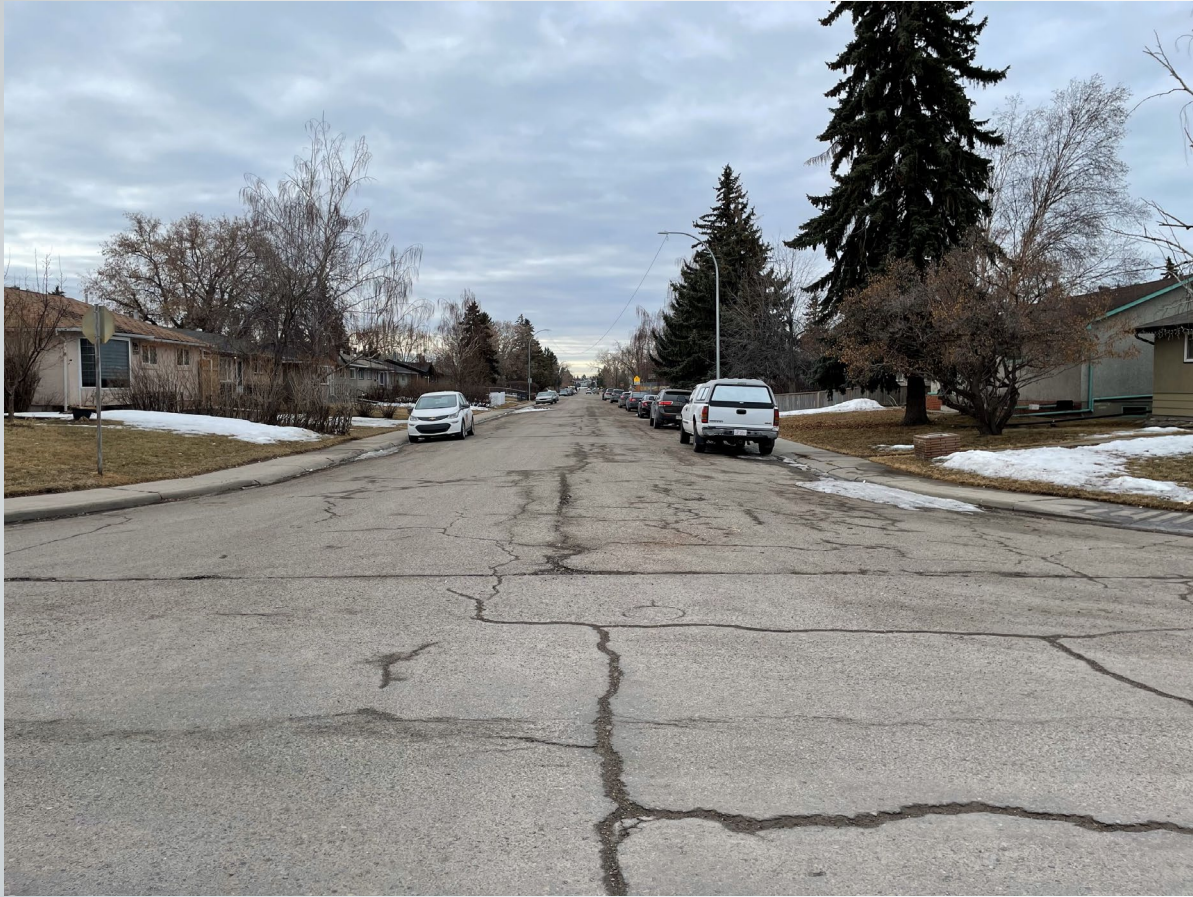
Looking south to 46 ST SE – immediate block context
