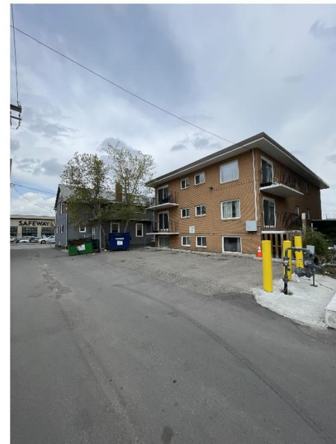
03. LANE LOOKING NORTH
