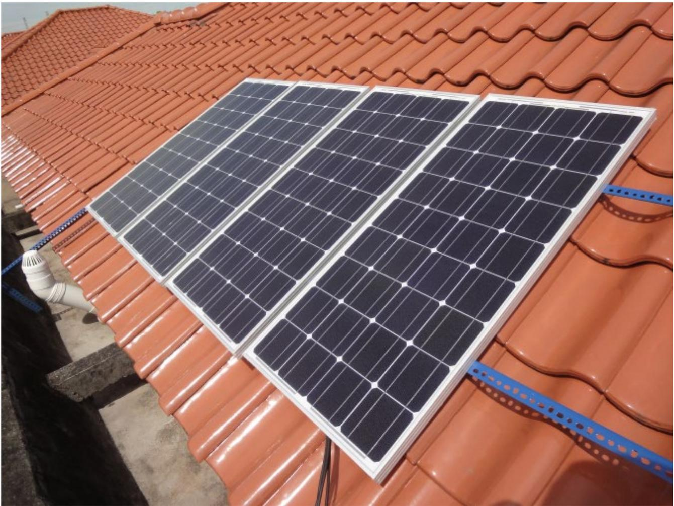
*Figure 1: A typical domestic solar array. Even a small shadow would result in the power output being reduced from the affected panels.*
