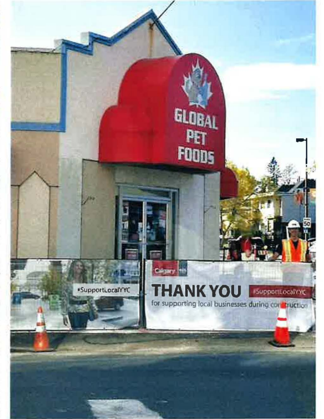
Marketing to encourage Calgarians to support local businesses during construction
