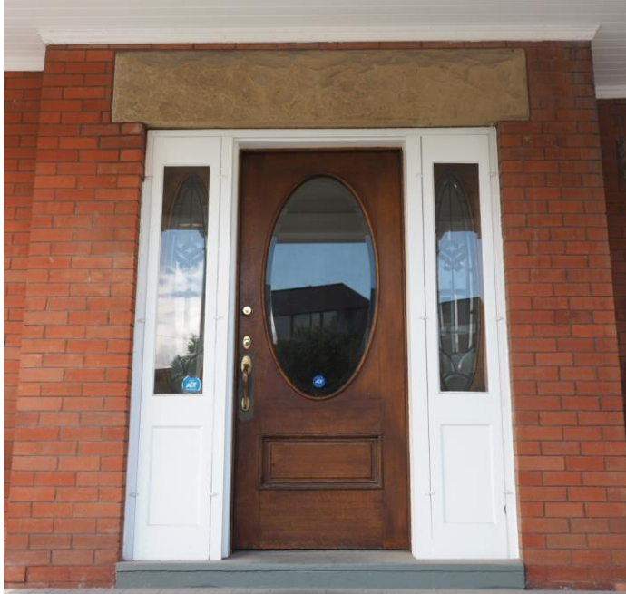
(Image 1.3 – Main entrance, showing doorway assembly)
