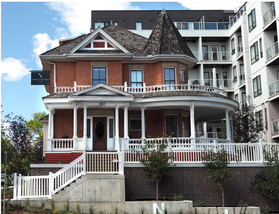
(Image 1.2 – East façade of the Nimmons Residence; contemporary L-shaped stair accessing veranda is non-regulated)
