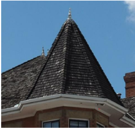
(Image 5.0 – Detail view of turret roof)
