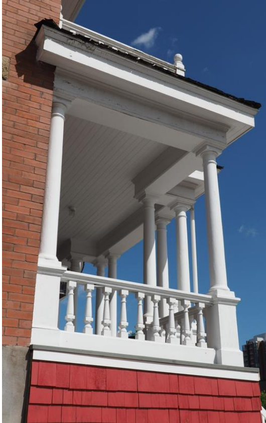
(Image 1.9 – South facade of the veranda, showing column detail and tongue-and-groove ceiling)
