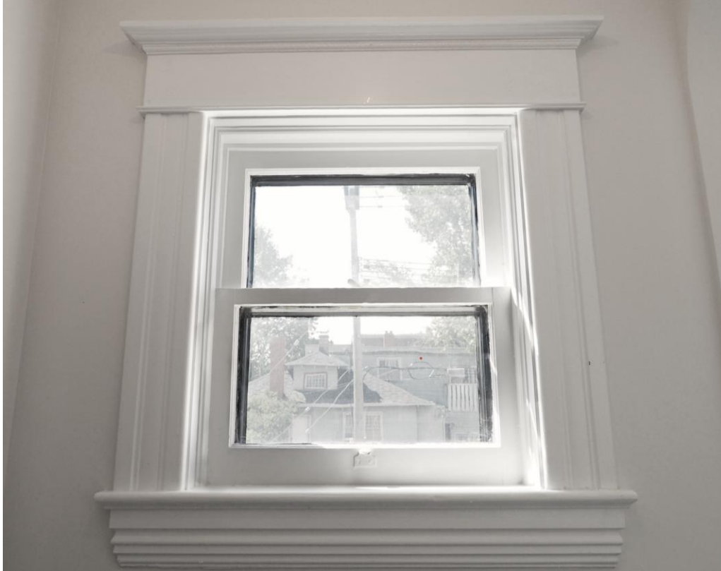
(Image 6.3 – Detail view showing more-ornate example of complete window casing)
