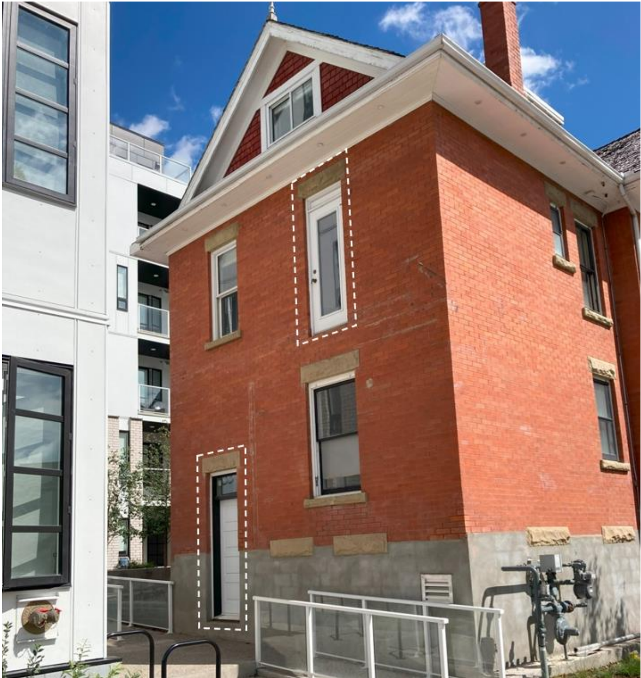
(Image 4.1 – Oblique view of the Nimmons Residence, looking northeast; dotted outlines indicate alterations to west façade from prior contemporary addition)
