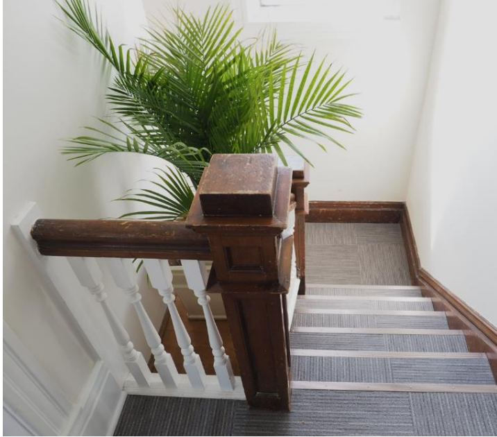
(Image 6.5 – Main staircase, looking from top of stairs, showing second-storey newel post)
