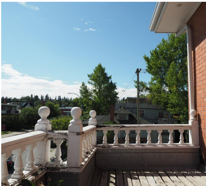
(Image 1.13 – Balustrade at balcony level, looking south)
