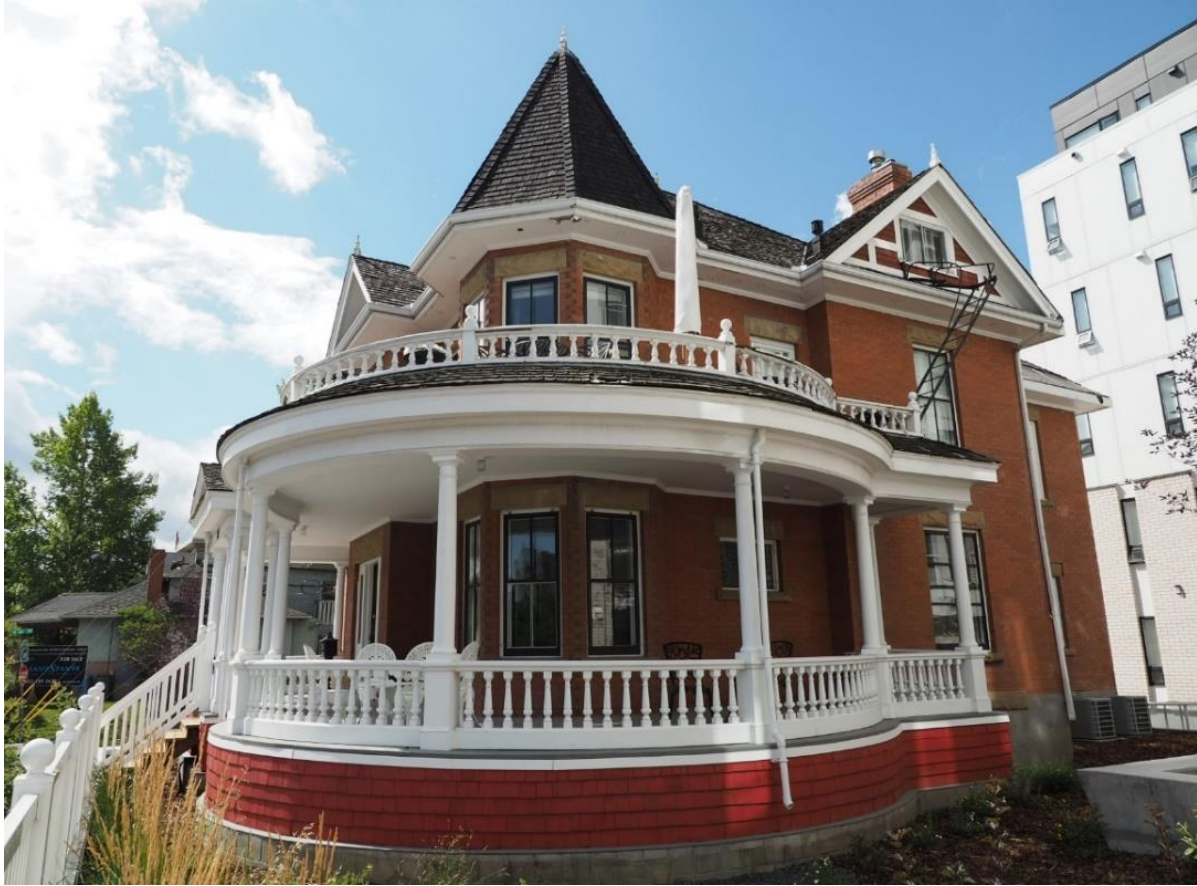
(Image 3.2 – Oblique view of the Nimmons Residence, looking southwest)
